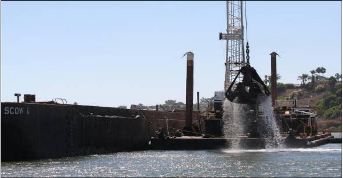
Clamshell Dredge with 5 cubic yard bucket and 3000 cubic yard scow, dredging Sediment Basin II.
