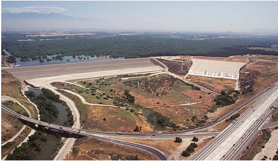
Figure 7-14: View to the North of Prado Dam (to the right-center), and Prado Dam Reservoir (in the Background)
