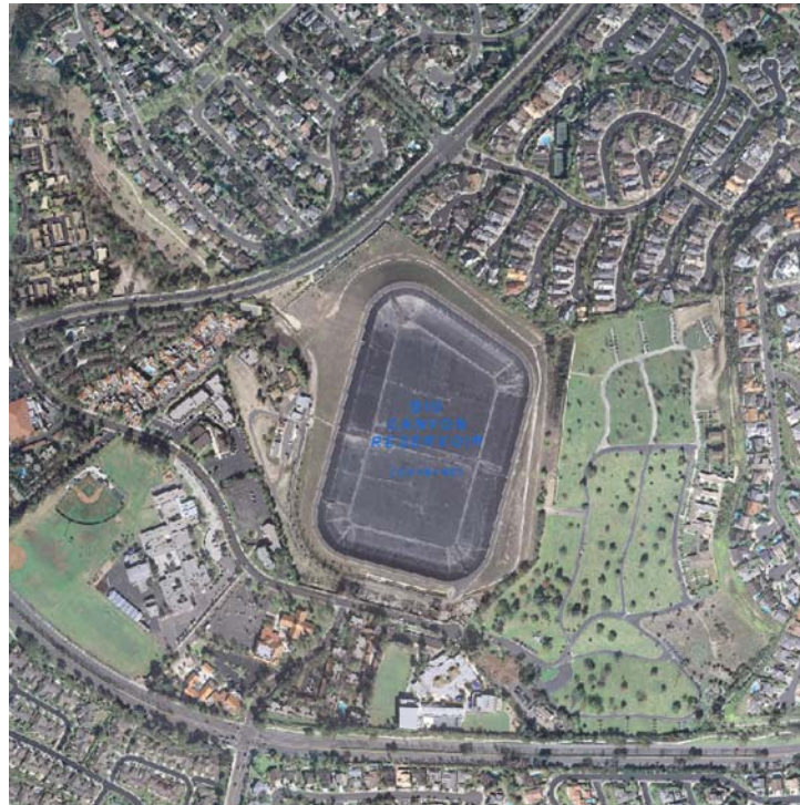
Figure 7-17: View of Big Canyon Dam and Reservoir (North to the top; photo courtesy of City of Newport Beach; December 2007)
