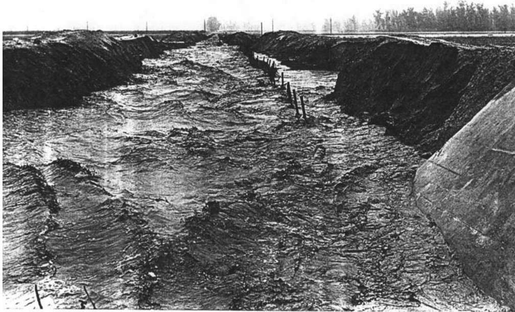
Figure 7-4: Photograph Looking Downstream at Flooding on Peters Canyon Wash (February 25, 1969)
