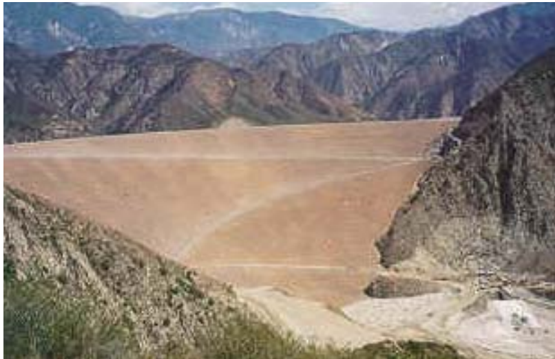
Figure 7-15: View Upstream of Seven Oaks Dam
