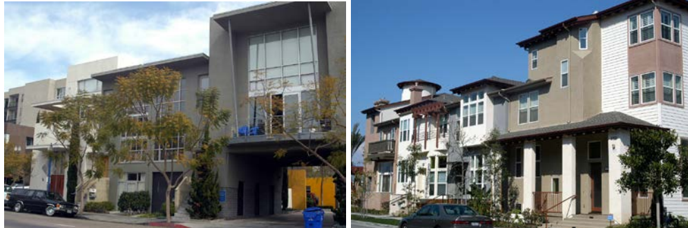
Illustrates multi-family residential with lobbies and entry gates located on each street and pedestrian-way frontage.
