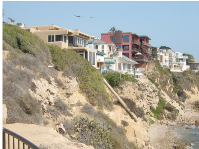
Coastal bluff erosion along the Newport Beach coastline
