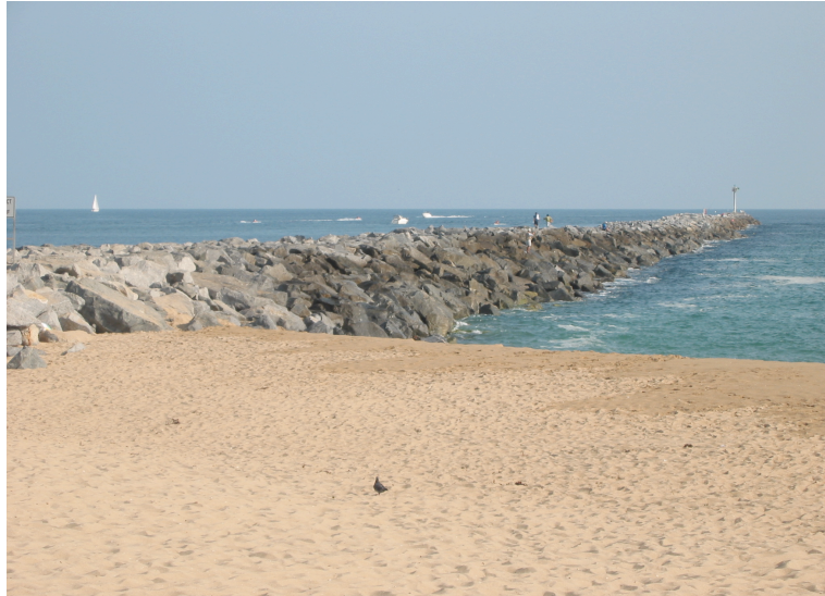
Figure 1-4: Artificial Coastal Protection; Rock Groin along Newport Beach
