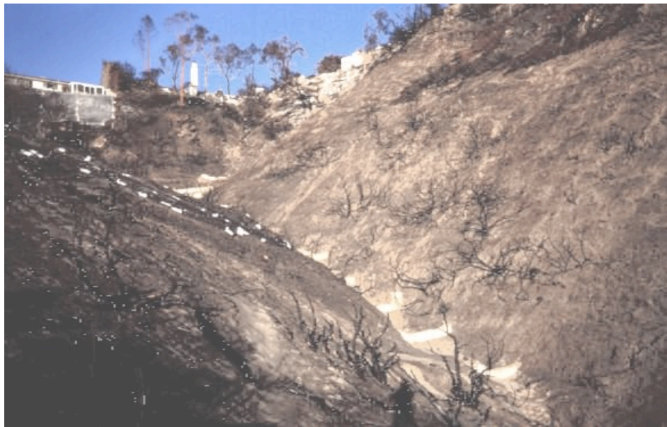
Figure 5-5: Photograph Showing Denudation of Slopes Following the 1993 Laguna Beach Fire. Sandbags, plastic covers and other measures were implemented as soon as possible to reduce the potential for slope instability during the winter following the fire.
