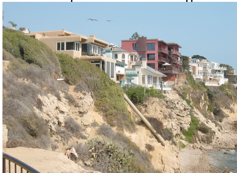
Figure 1-3: Near-Bluff Development and Erosion of Slopes due to Increased Water Application
