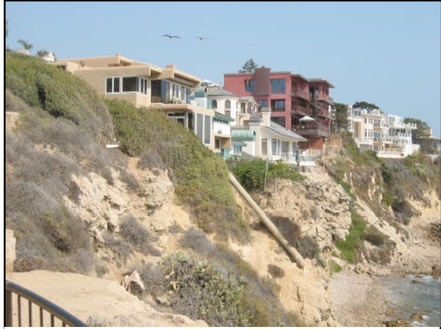
Erosion of coastal bluffs due to increased water application
