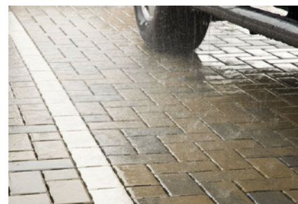
Vehicular Pavers and Striping
