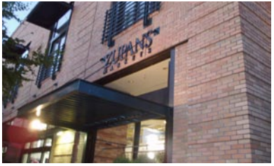
Metal Awning Shelters Entrance
