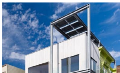
Integrated Solar Panels
