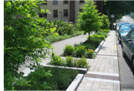
'Green Street' Bio-swale
