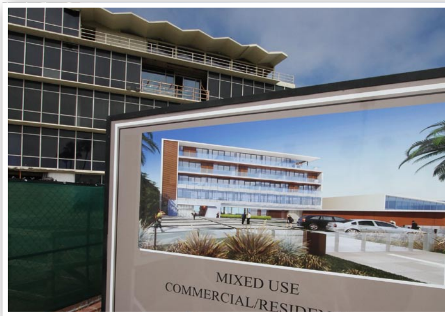
Renovations Underway within Lido Village
