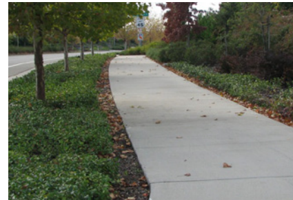
A 'clear edge' to aid in maintenance and minimize over-spray
