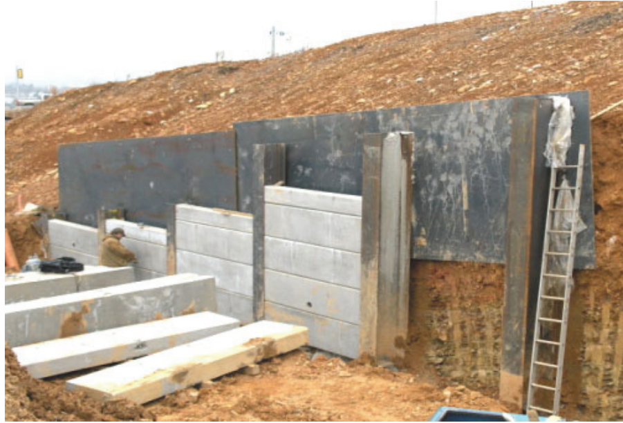
Figure 5.4 Construction of Retaining Wall Using H-piles and Concrete Wall (Lag) Panels
