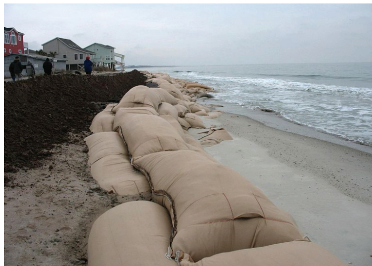
Figure 5.1 Geotextile Sandbags Used as a Seawall Along a Beach
