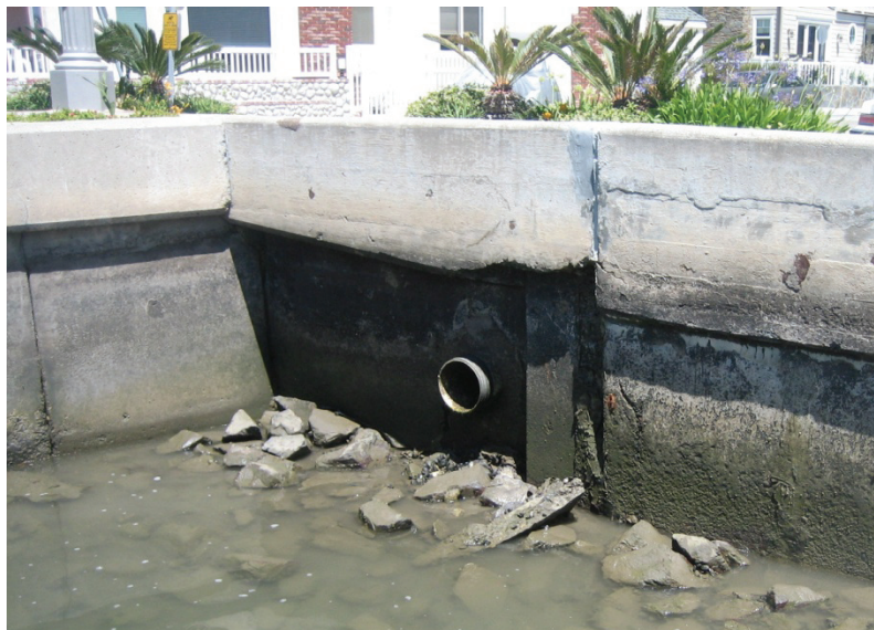
Figure 4.9 Storm Drain Outlet Through Seawall
