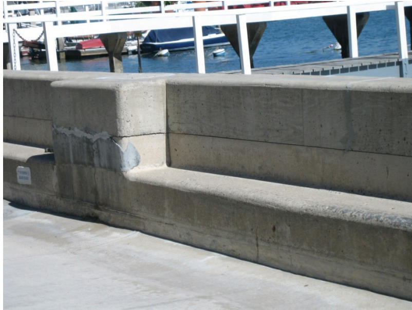
Figure 4.4 Little Balboa Seawall Cap Extension
