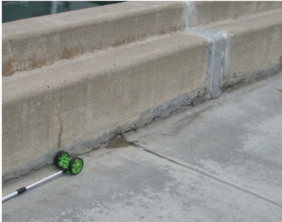
Figure 4.8 Sidewalk Separation from Seawall
