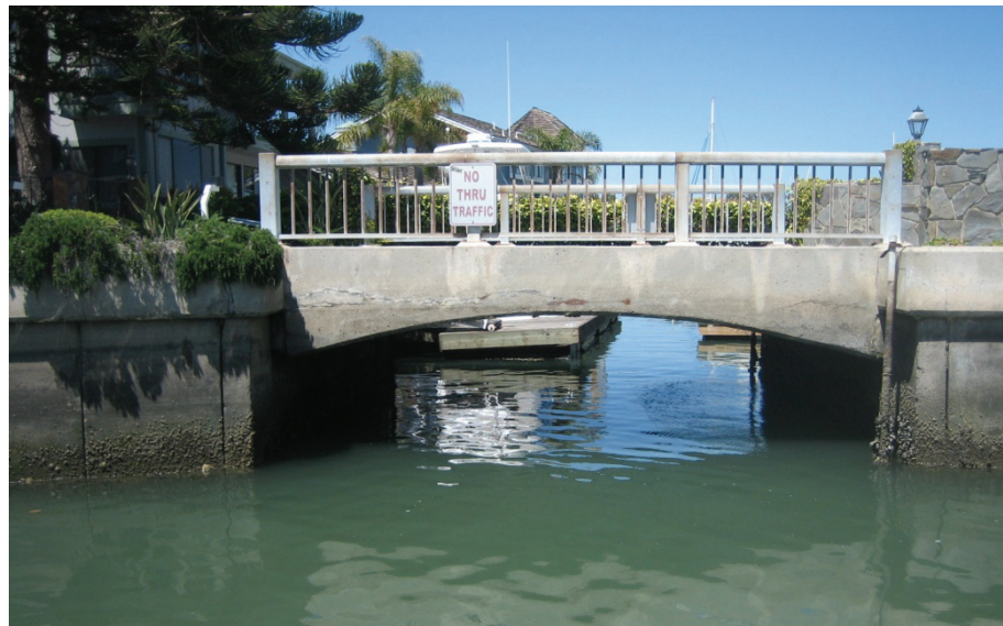
Figure 4.13 Collins Island Bridge Interface at Seawall Abutment
