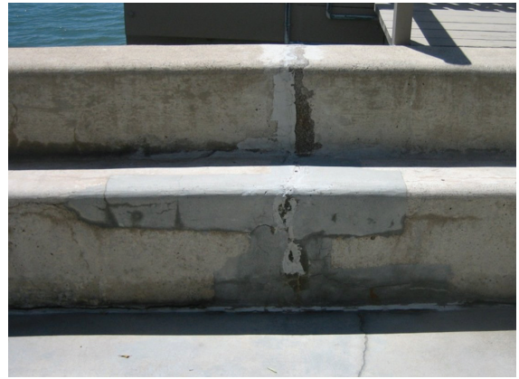
Figure 4.6 Typical Crack and Spall Repairs
