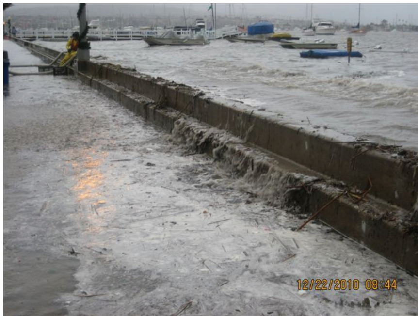
Figure 1.4 Bay Waters Overtopping the Seawall
