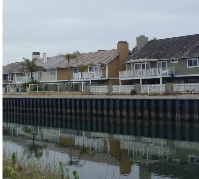
Figure 5.6 Steel Sheet Pile Bulkhead
