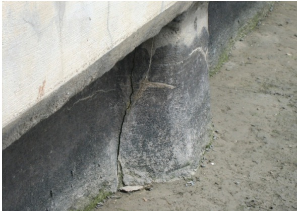
Figure 4.5 Shot-crete on Grand Canal Seawall
