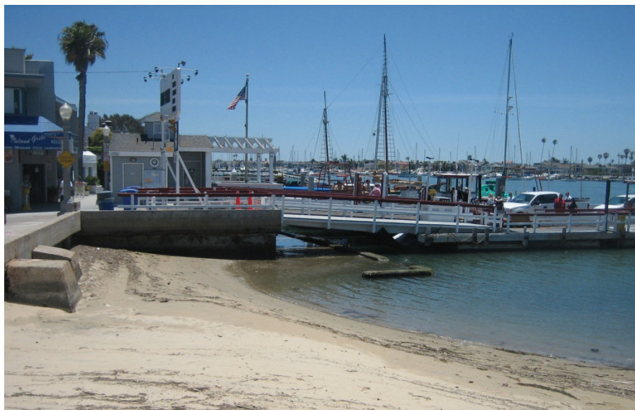
Figure 4.15 Balboa Island Ferry Boat Landing as Viewed from Side
