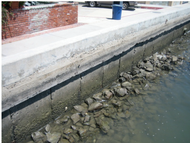
Figure 4.1 Rock Revetment Stabilization at Western End of Balboa Island
