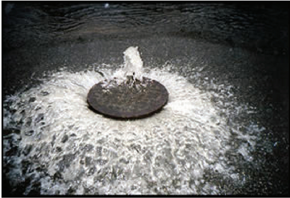
Figure 1.1 Example of a Sanitary Sewer Overflow
