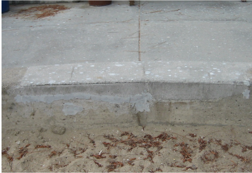
Figure 4.3 Use of Elastomeric Filler to Seal Cracks to Prevent Seawater Intrusion
