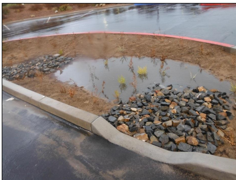
Figure 3-8. West Bioretention BMP during October 9, 2013 Storm Event
