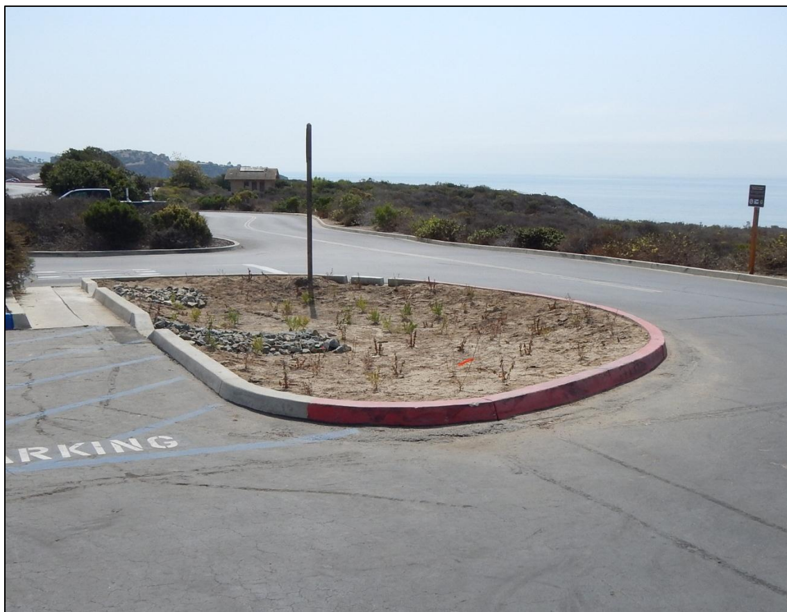
Figure 1-2. Southwest Bioretention Planter BMP
