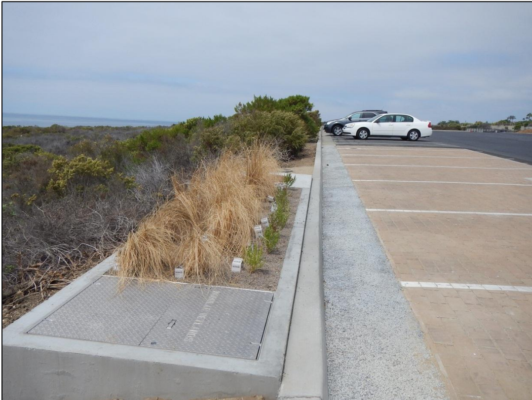
Figure 1-3. Porous Pavers and Modular Wetland System Treatment BMPs
