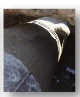
Once the relining was complete, Water Maintenance and Repair staff cut out the damaged section of the water main and welded on a steel strap. Before backfilling, staff covered the pipe with protective tape and coated it with concrete to protect the steel from elements that could accelerate corrosion.
