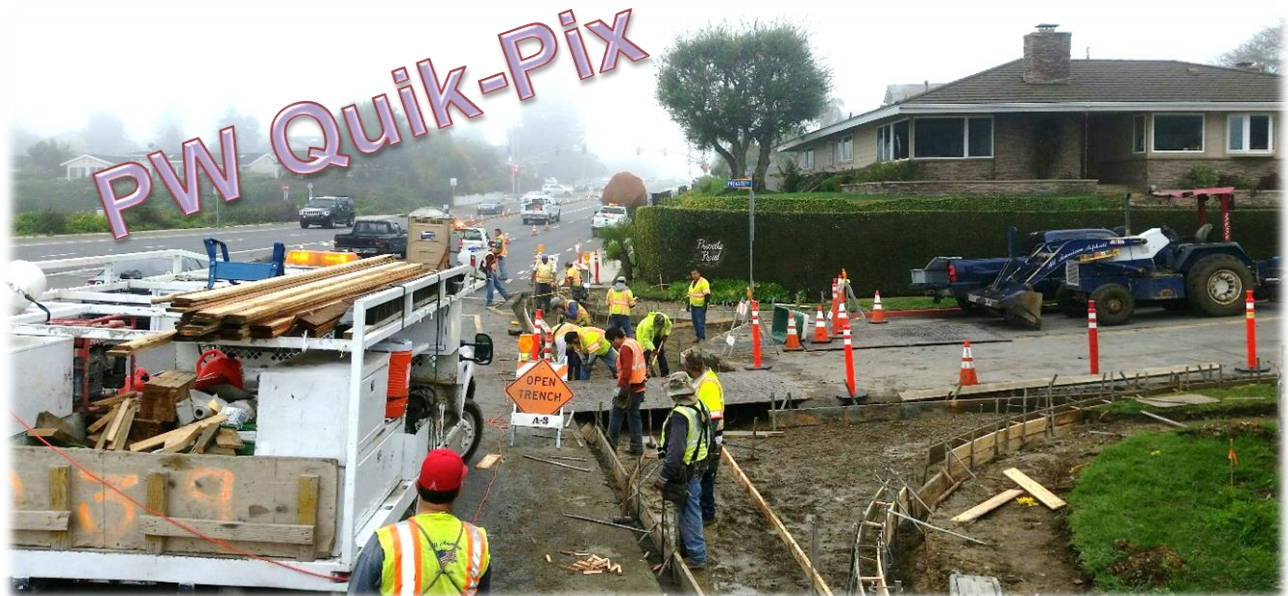
Crews Preparing to Pour Concrete for New Cross Gutter at Irvine Avenue & Private Road
