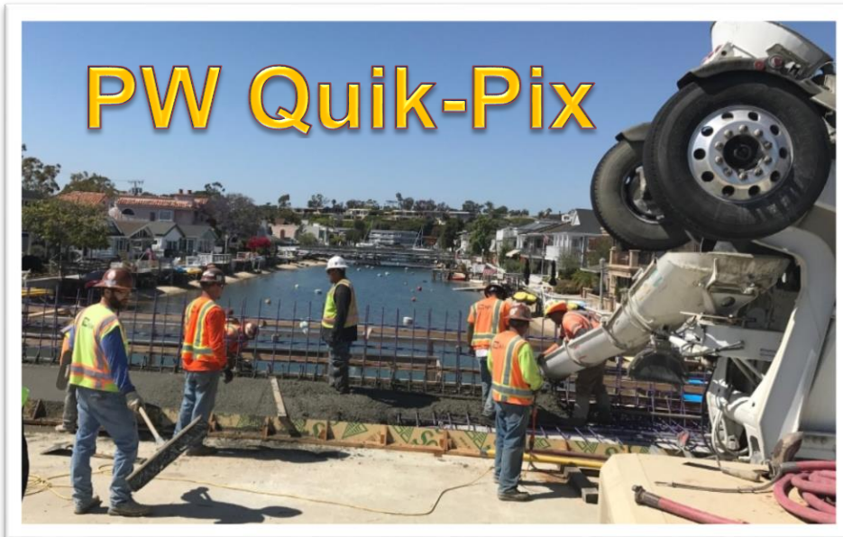
Pictured At Left: Park Avenue Bridge Sidewalk Concrete Pour
