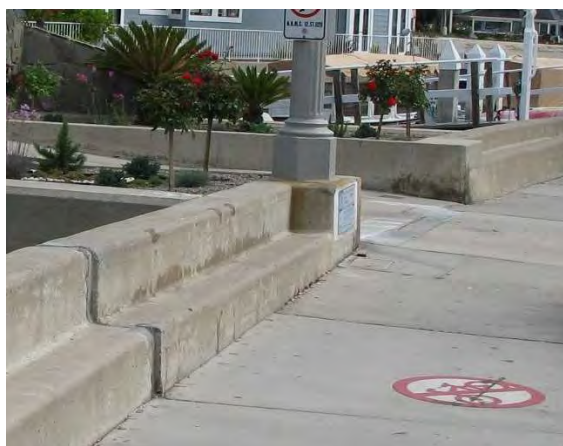
Photo 10 – Offset in wall at change in bulkhead construction. Station S+74
