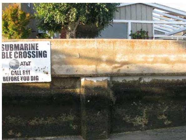
Photo 9 – Photo showing flexible sealant present in some locations, but not all.
