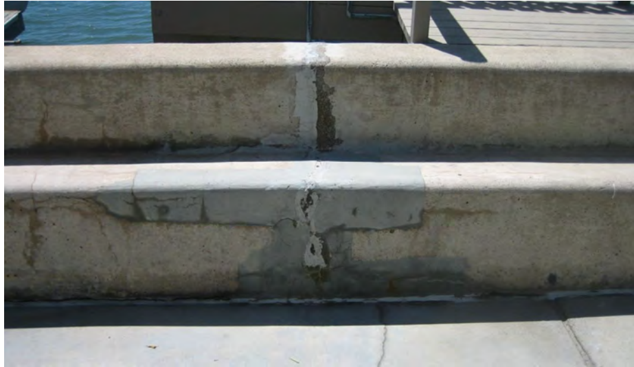
Photo 11: Typical spall and crack repairs
