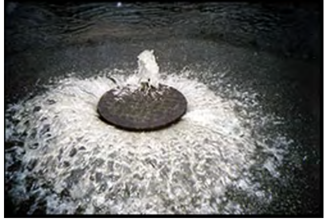
Photo 33: Example of Sanitary Sewer Overflow
