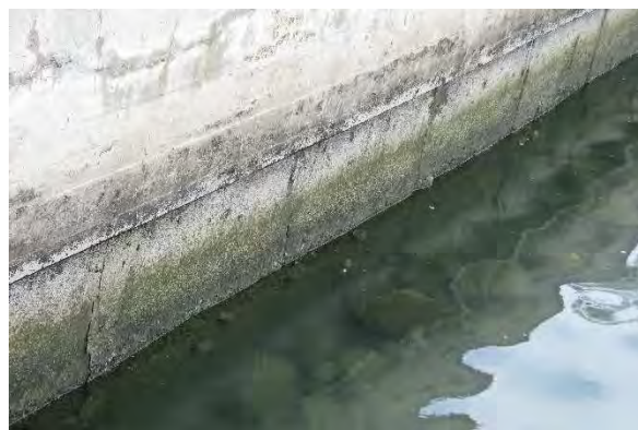
Photo 6 – Typical cementitious precast panel joint sealing south of Collins Island Bridge
