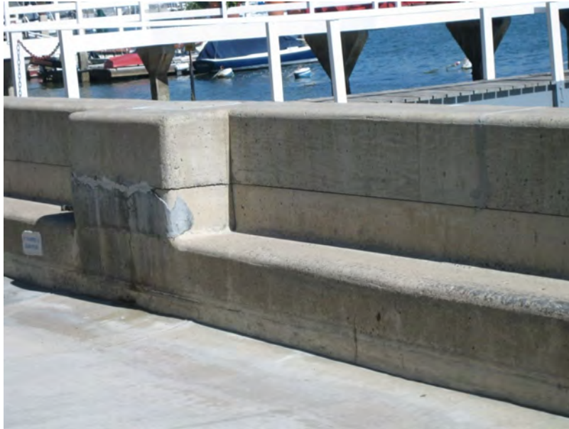
Photo 9: Little Balboa seawall cap extension
