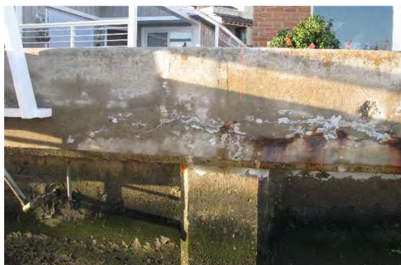
Photo 8 - Major cracking over soldier pile, with rust staining and previous repair. Station N2+70
