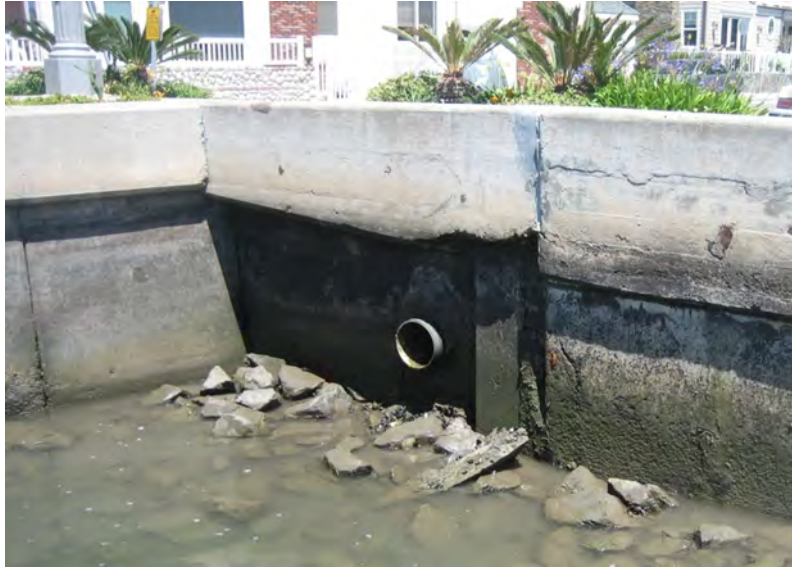
Photo 19: Storm drain outlet through seawall
