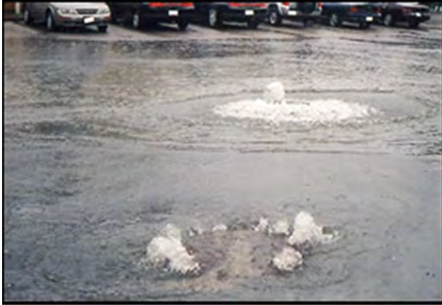
Photo 32: Example of Sanitary Sewer Overflow
