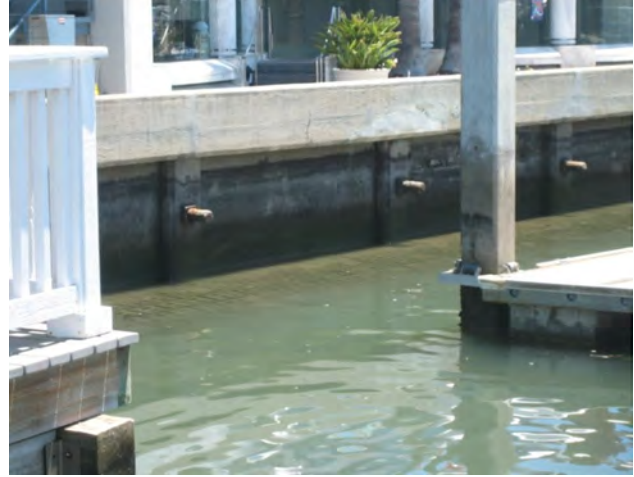
Photo 2: Earth anchors and concrete block revetment (submerged) at Balboa Island Ferry Boat Landing
