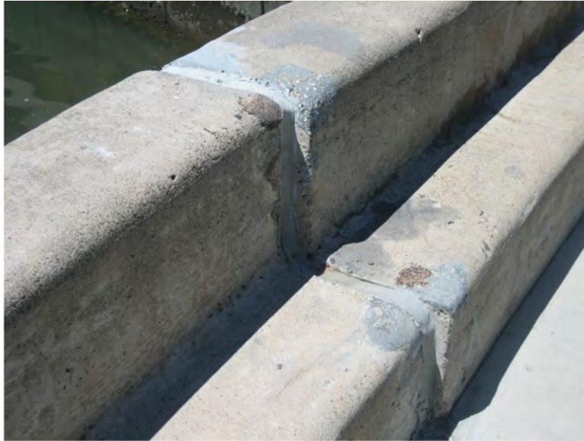
Photo 4: Use of elastomeric filler at joint
