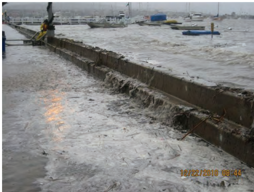
Figure 1.4 Bay Waters Overtopping the Seawall
