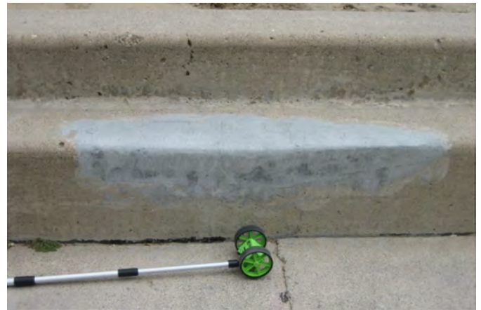
Photo 12: Successful spall repairs
