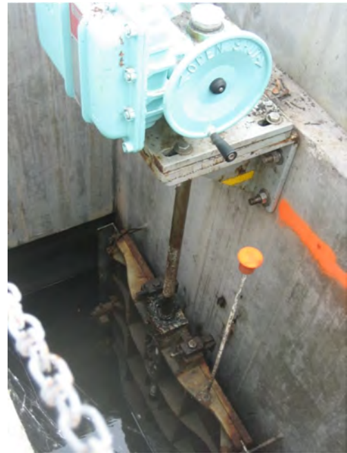
Photo 21: Actuated gate valve in storm drain vault
