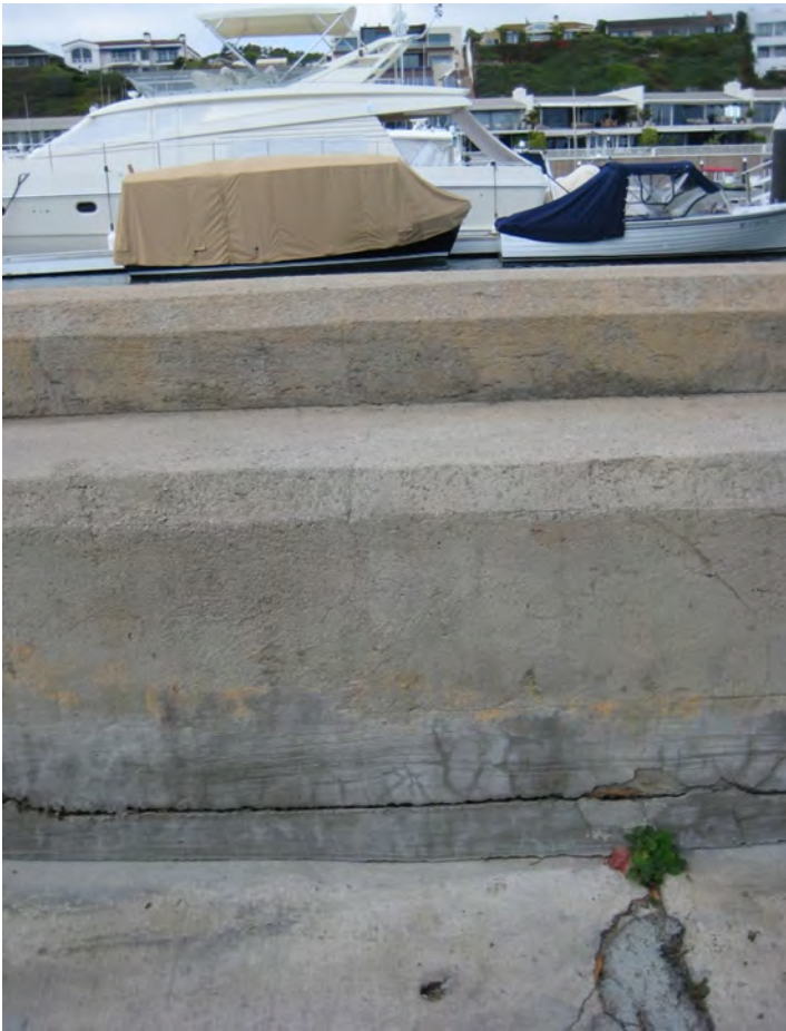
Photo 14: Crack along sidewalk separation from seawall
