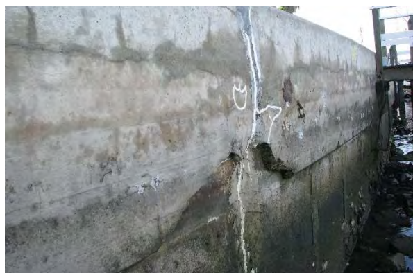
Photo 5 – Coping spalled, both sides, above precast wall panel joint. Joint previously sealed with cementitious grout and flexible sealant. Station S3+62
