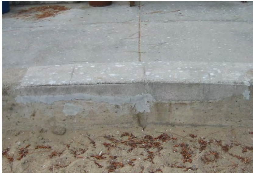
Photo 3: Use of elastomeric filler to seal cracks to prevent seawater intrusion
