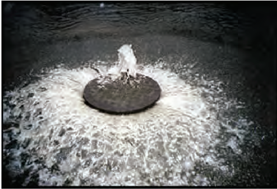
Figure 1.1 Example of a Sanitary Sewer Overflow
