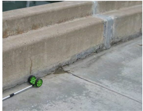
Photo 15: Sidewalk separation from seawall
