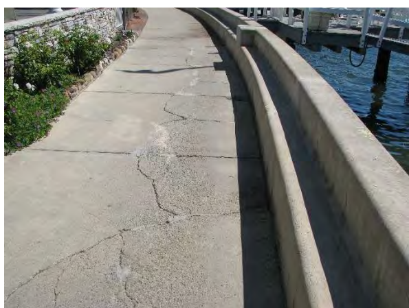
Photo 10 – Major cracks in sidewalk. Station S4+21
