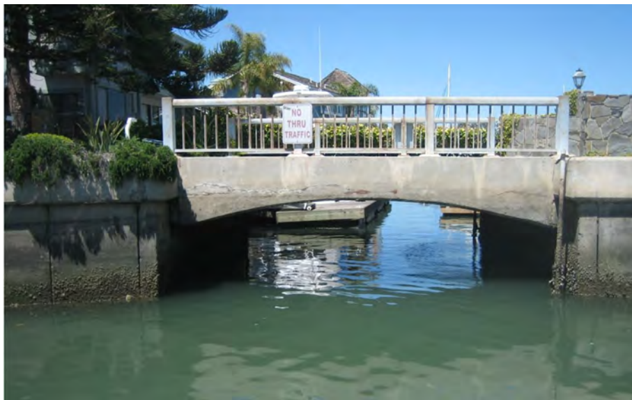
Photo 27: Collins Island Bridge interface at seawall abutment
