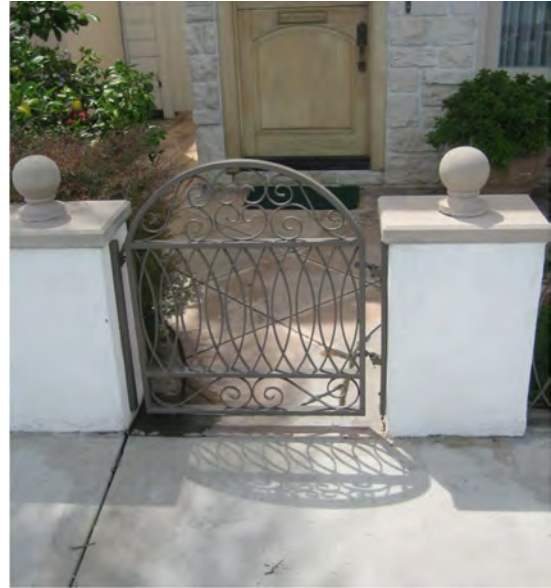
Photo 6: Residential finish floor transition to sidewalk
