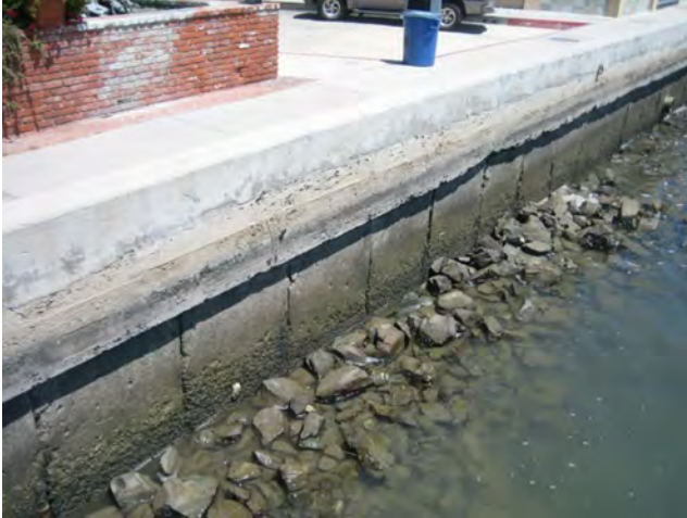
Photo 1: Rock revetment stabilization at western end of Big Balboa Island
