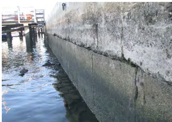
Photo 2 – Erosion of wall and coping from station S0+09 to S0+31
