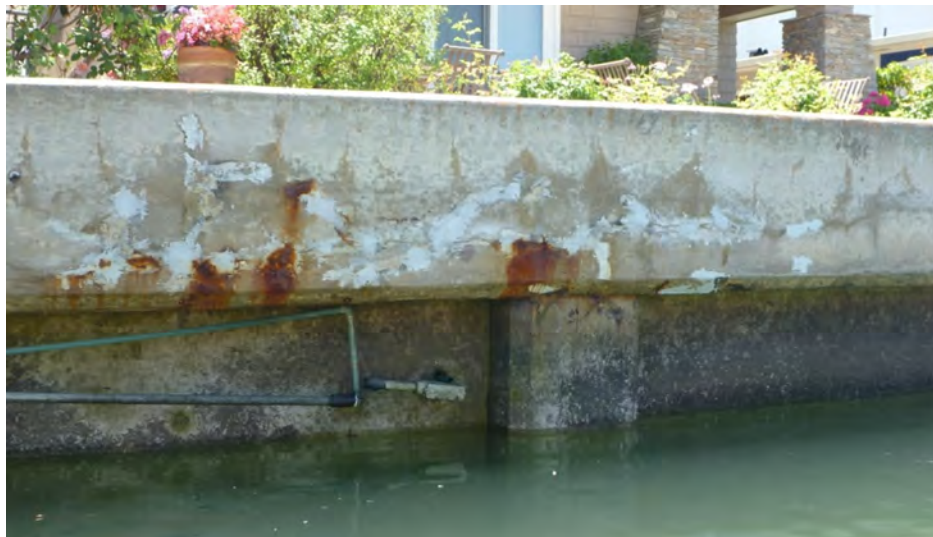
Photo 13: Crack repairs with corroding rebar
