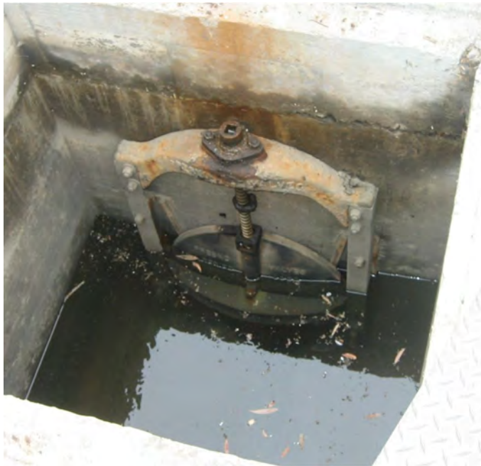
Photo 20: Hand-operated gate valve in storm drain manhole
