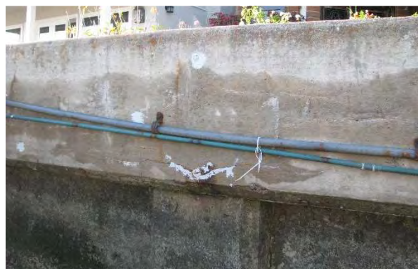
Photo 7 – Minor to Moderate cracking over soldier pile, with partial previous repair. Station N1+54
