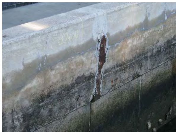
Photo 3 – Previous cementitious repair exhibiting rust stains at bent S2+92
