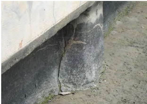
Photo 10: Shot-crete on Grand Canal seawall
