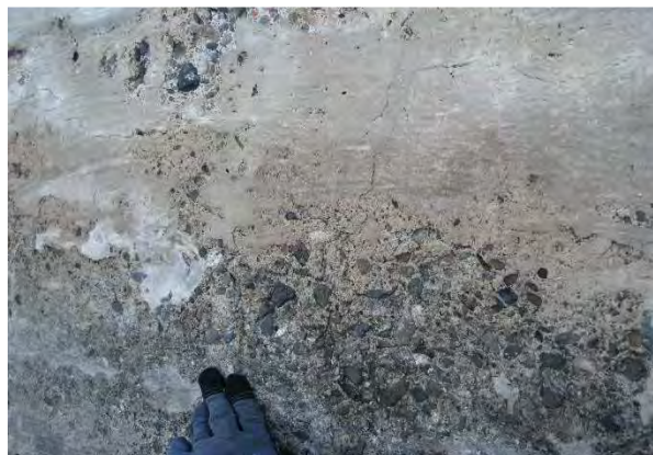
Photo 1 – Example of hairline cracks, not individually called out in defect tables
