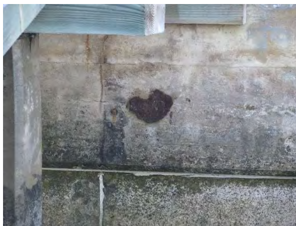
Photo 4 – Rusted plug at wall, with flexible sealant at joints, at station S3+08
