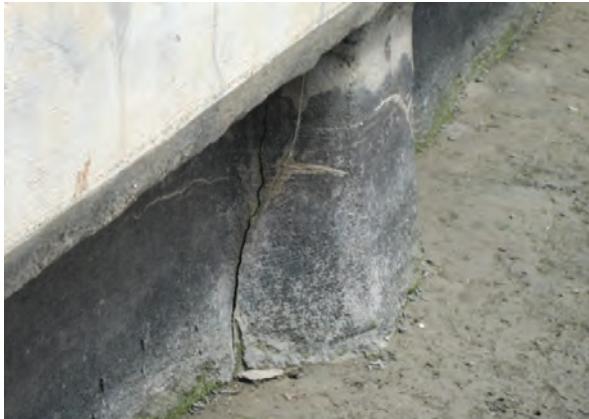
Figure 4.5 Shot-crete on Grand Canal Seawall
