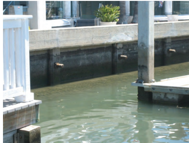
Figure 4.2 Earth Anchors and Concrete Block Revetment (Submerged) at Balboa Island Ferry Boat Landing
