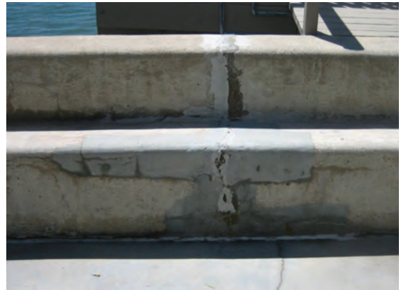
Figure 4.6 Typical Crack and Spall Repairs
