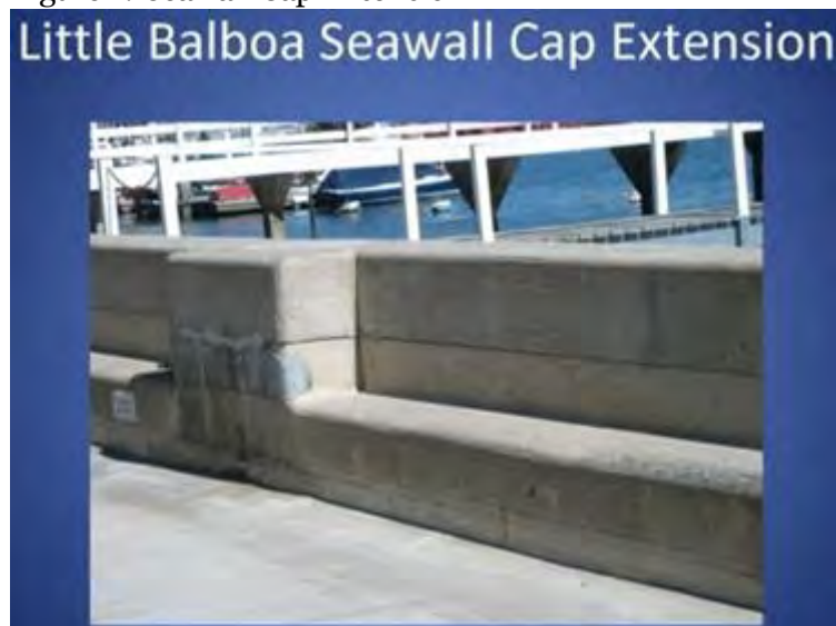
Figure 1: Seawall Cap Extension
