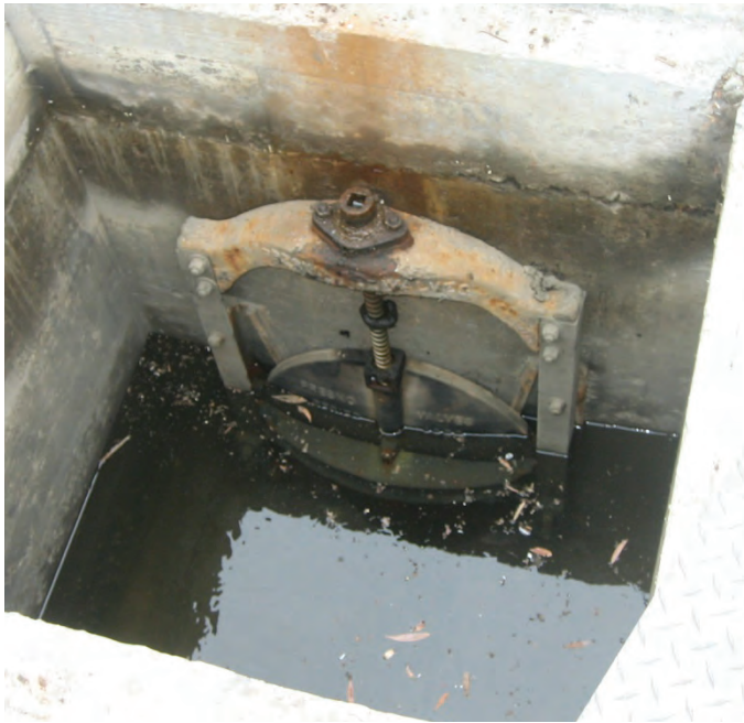
Figure 4.10 Hand-Operated Gate Valve in Storm Drain Manhole
