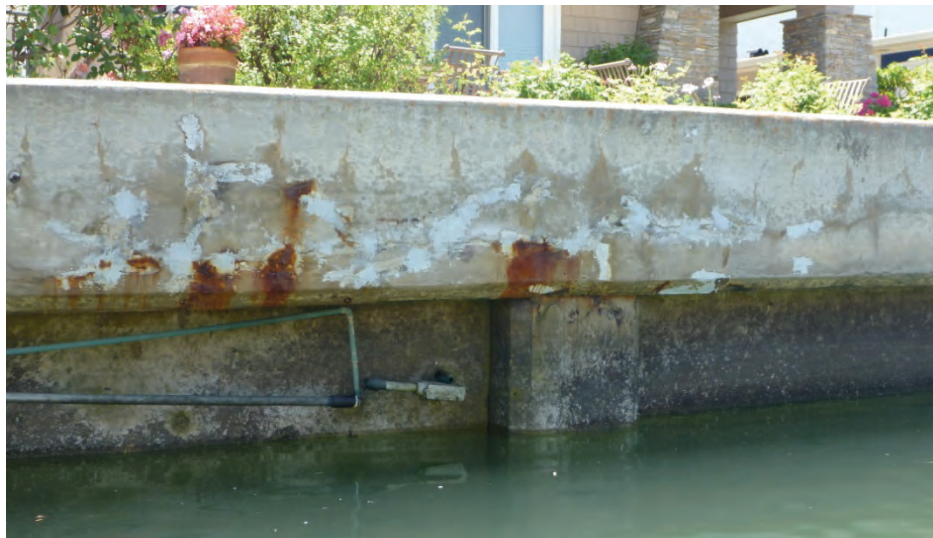
Figure 4.7 Crack Repairs with Corroding Rebar
