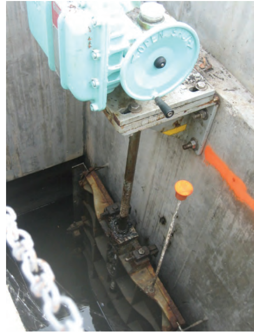
Figure 4.11 Actuated Gate Valve in Storm Drain Vault
