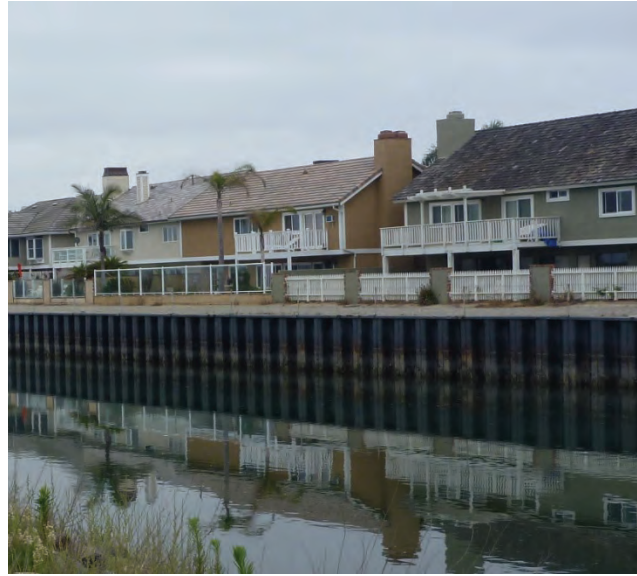
Figure 5.6 Steel Sheet Pile Bulkhead
