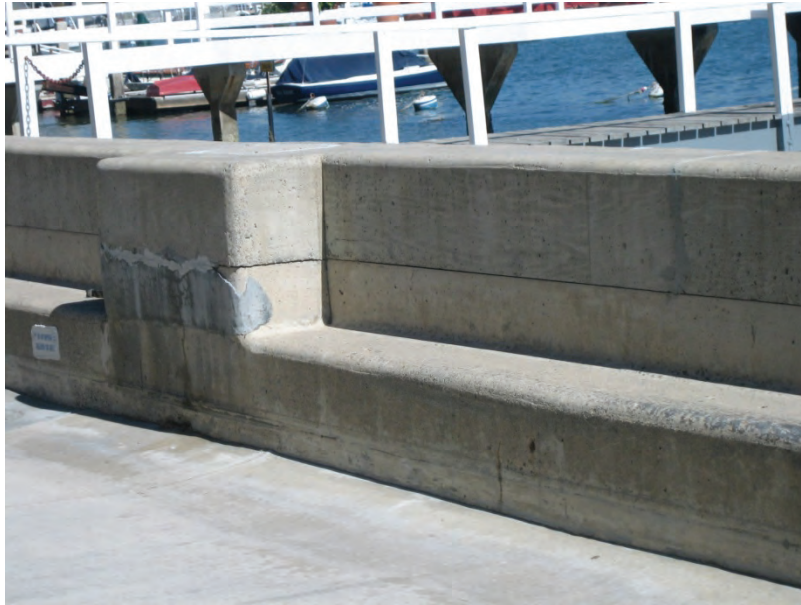
Figure 4.4 Little Balboa Seawall Cap Extension
