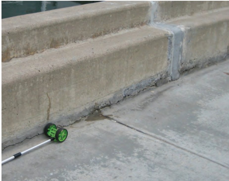
Figure 4.8 Sidewalk Separation from Seawall
