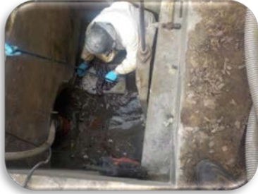
Injecting the sealant
