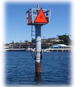
Current Steel Pile Marker
