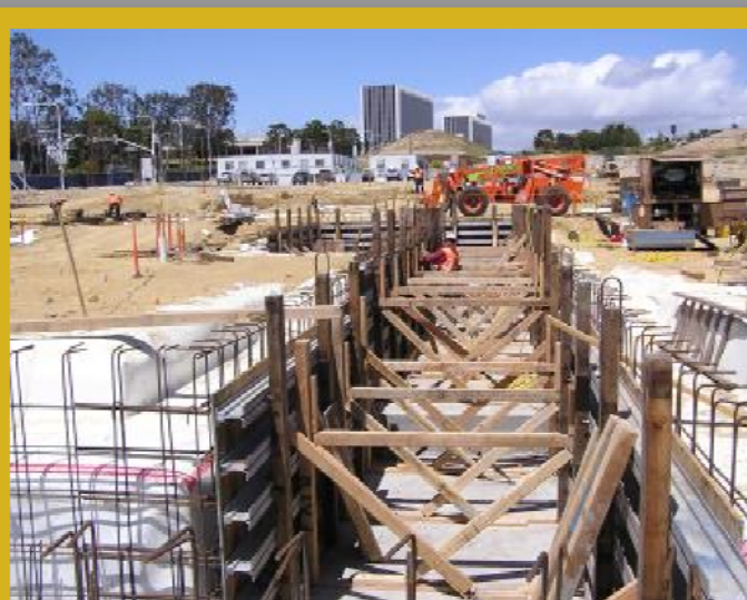
Forms for the city hall office building foundation
