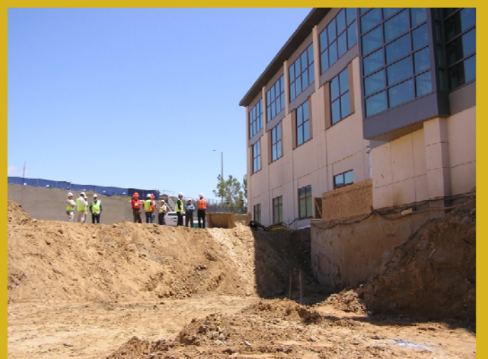
Future area for library expansion
