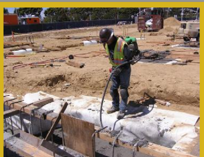
Verifying concrete compaction
