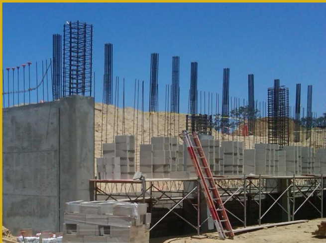
Parking structure support columns
