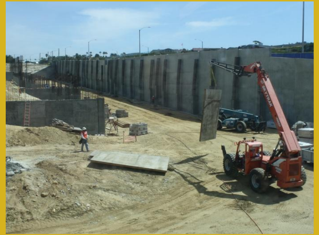
View from library second floor windows
