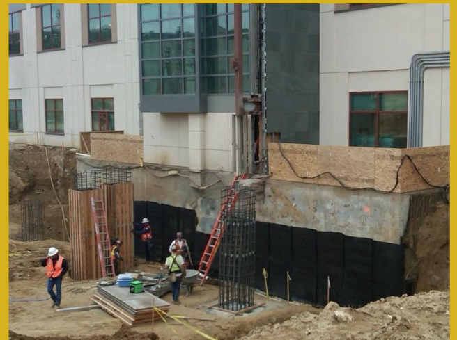
Waterproofing existing library foundation
