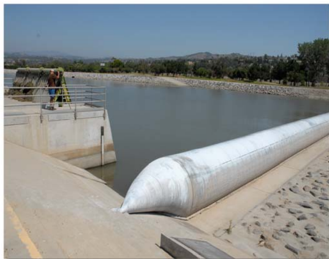
FIGURE 4-4 INFLATABLE DAM ON THE SANTA ANA RIVER
