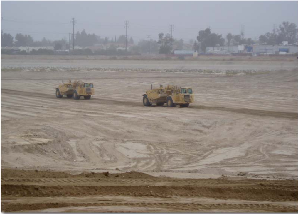
FIGURE 4-6 CLEANING OF RECHARGE BASINS
