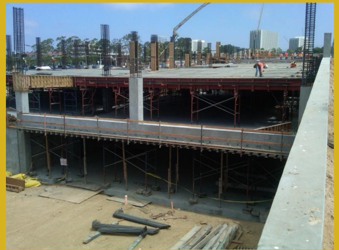
Parking structure view from the library
