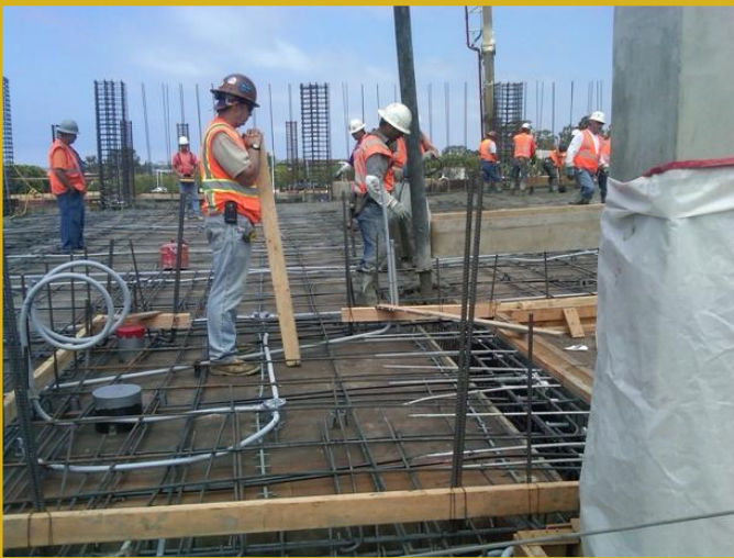
Preparing the parking structure's second floor for the concrete pour
