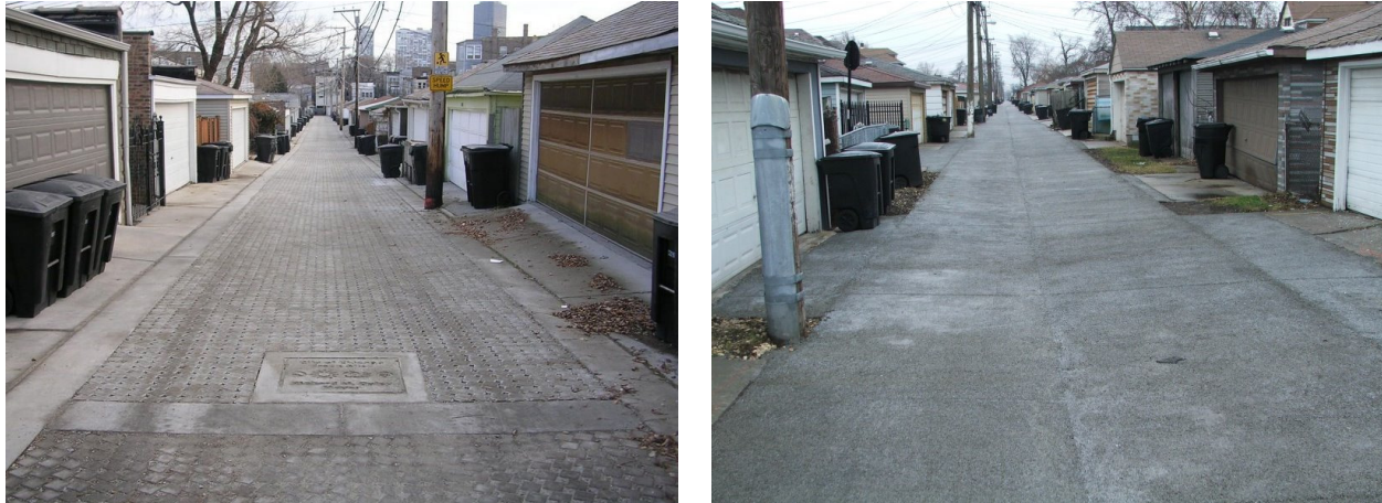
Figure 10: Permeable Pavers and Permeable Concrete Chicago Alleys (Source: Abby Hall, US EPA)
