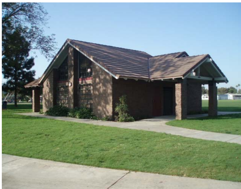
New Restrooms at Mariners Park
