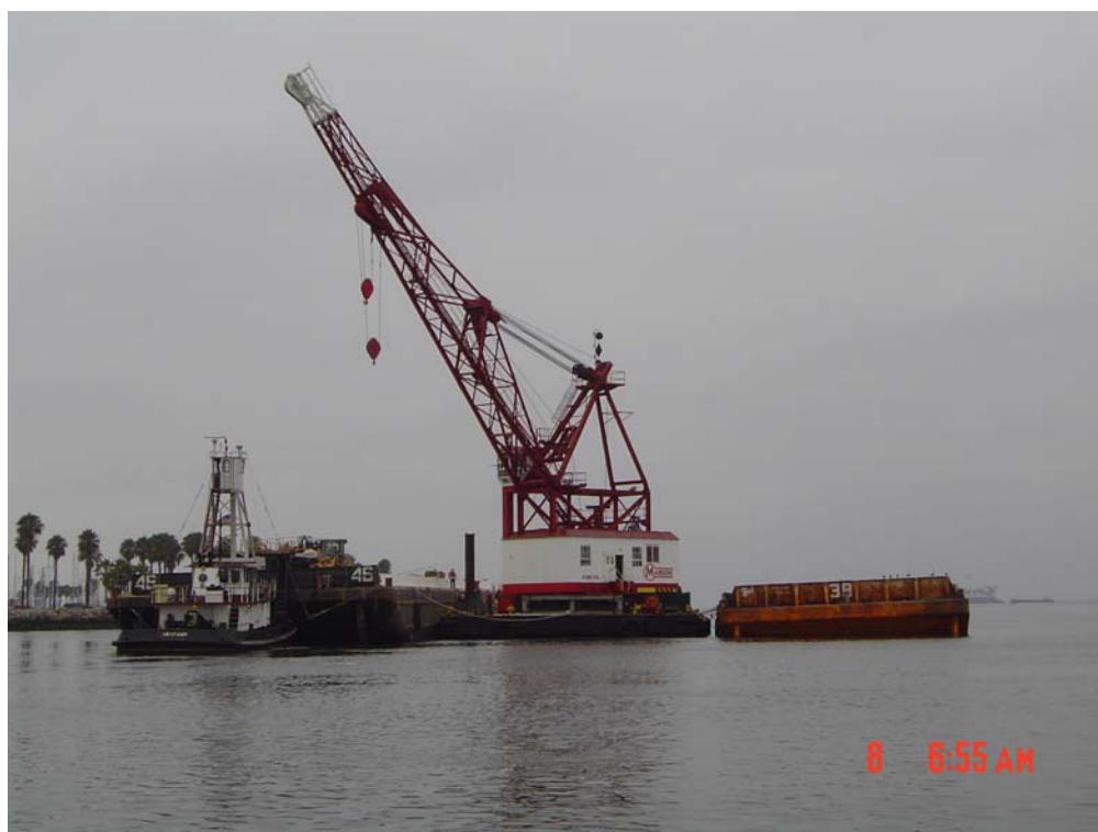
Figure C-3 Field Pilot Study Barge Layout (treatment equipment on left, derrick barge in middle and dredge material on right)
