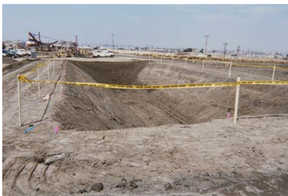
Photo B2-2. Completed and Secured Cell
