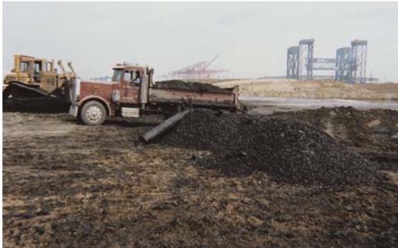
Photo B2-4. Dredged Material Placement into Treatment Cell
