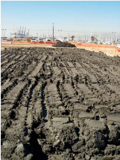
Photo B2-18. Disked Compaction Layer
