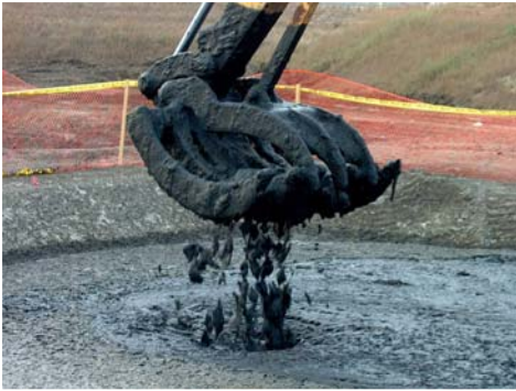
Photos B2-5A. Debris Removal
