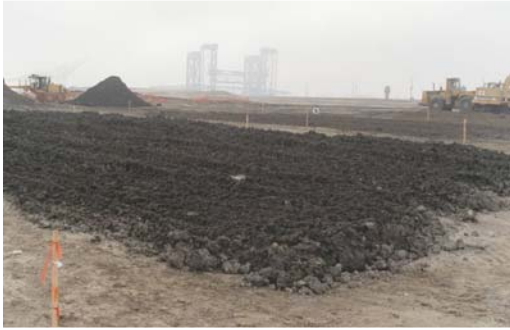
Photo B2-17. Initial Lifts of Compaction Pad
