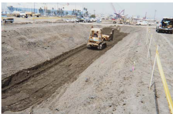
Photo B2-1. Treatment Cell under Construction
