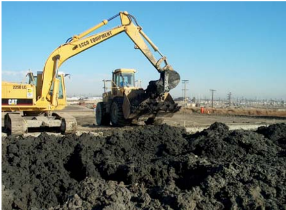
Photo B2-15. Excavation and Transfer of Treated Material for Stockpiling
