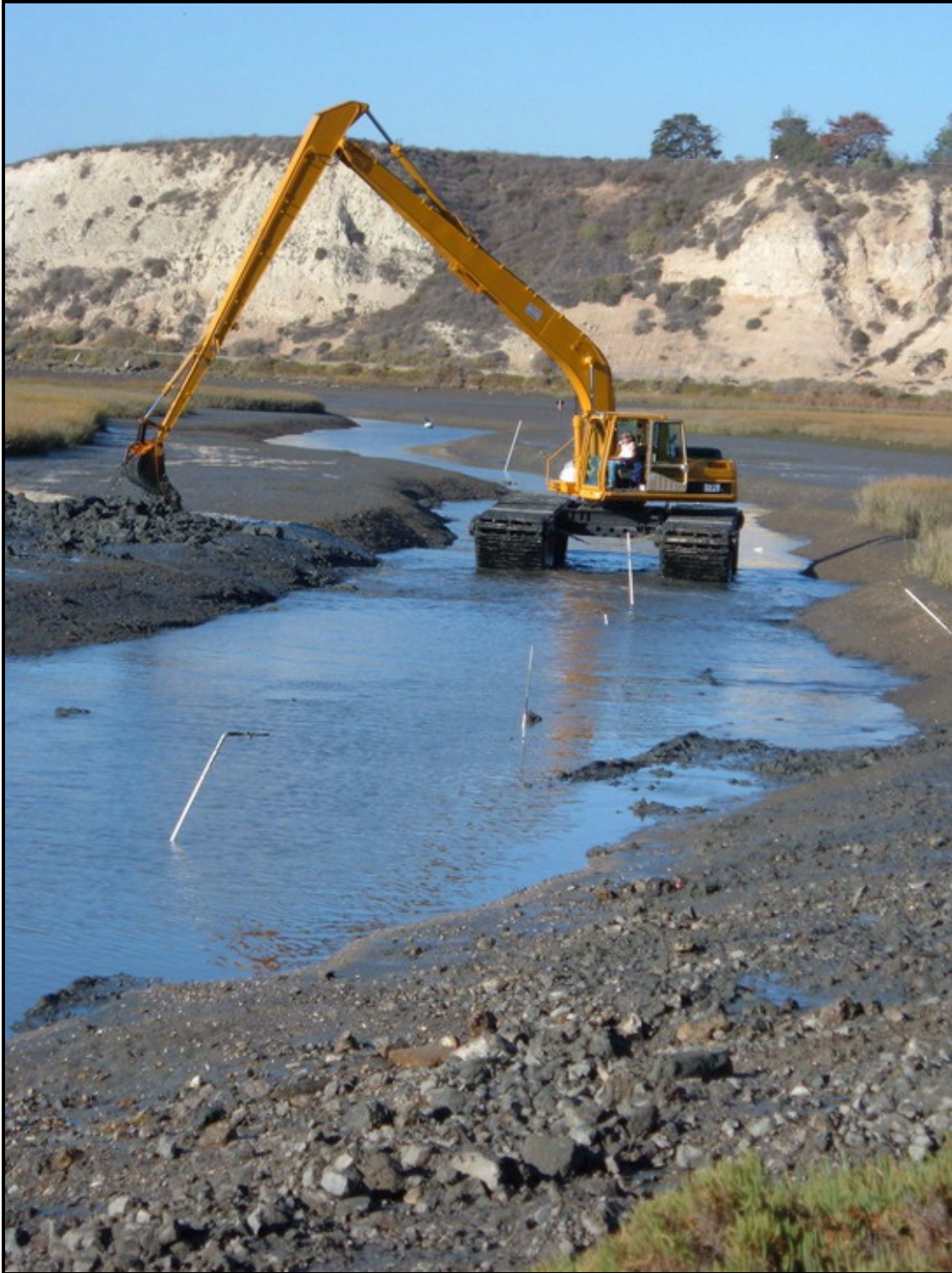
Amphibious Excavator working in Shellmaker Island, October 2008
