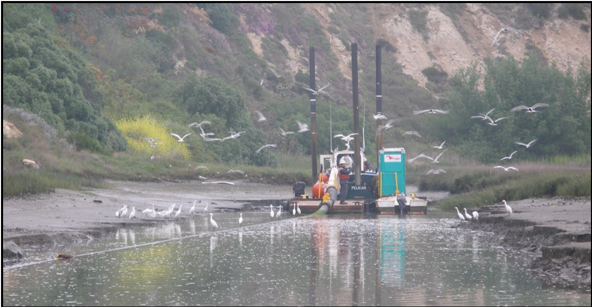
Hydraulic Dredge "Pelican" dredging Middle Island Restoration Channel, May 2006
