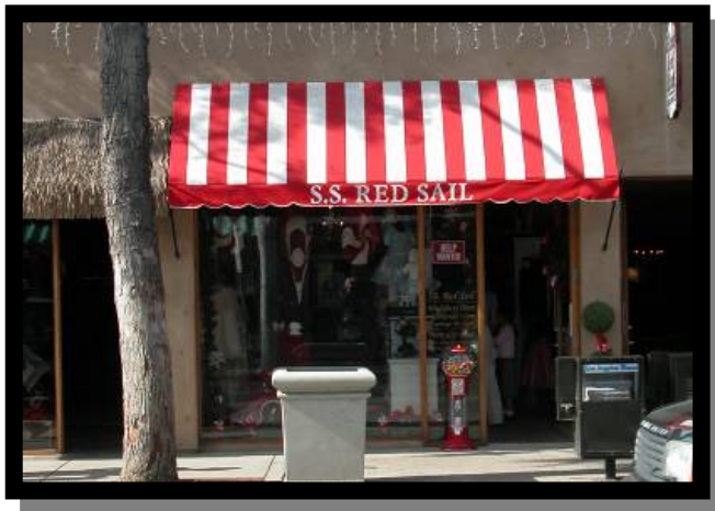
Good example of awning shape coordinated with window size/shape.
