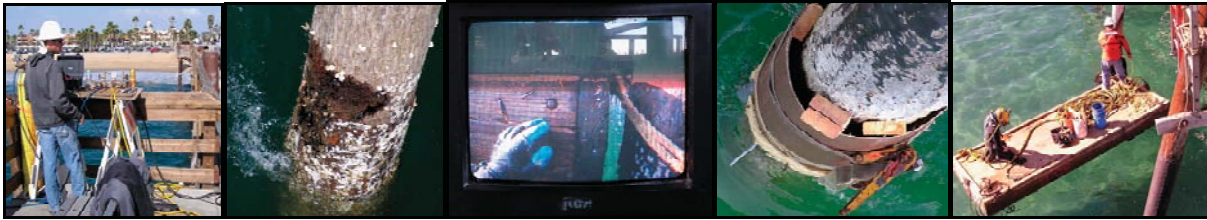
Ocean Pier Repair
