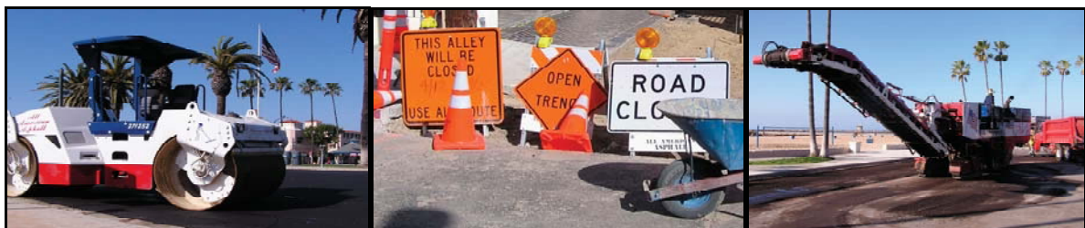
Citywide Paving and Parking Lot Rehabilitation
