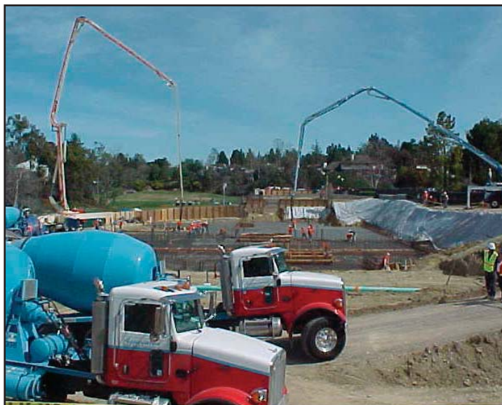
Concrete placement for the new Big Canyon Country Club Foundation
