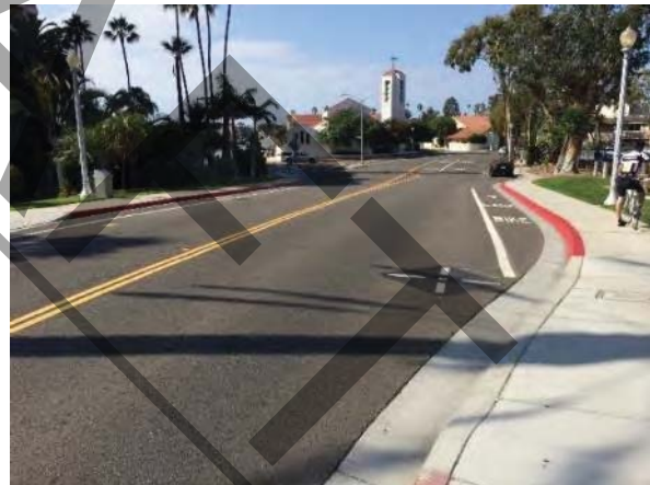
Bike lane on the west side of the Via Lido Bridge
