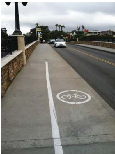
Striping on the south side of the Marine Avenue bridge
