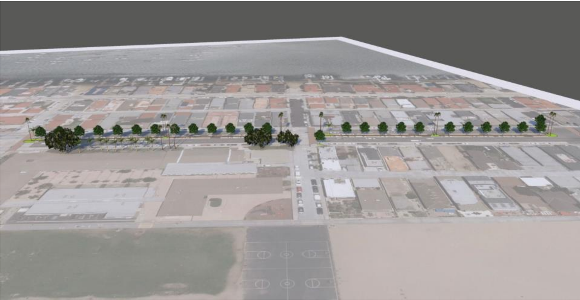
Aerial view of W. Balboa Blvd., 14 th Street to 12 th Street
