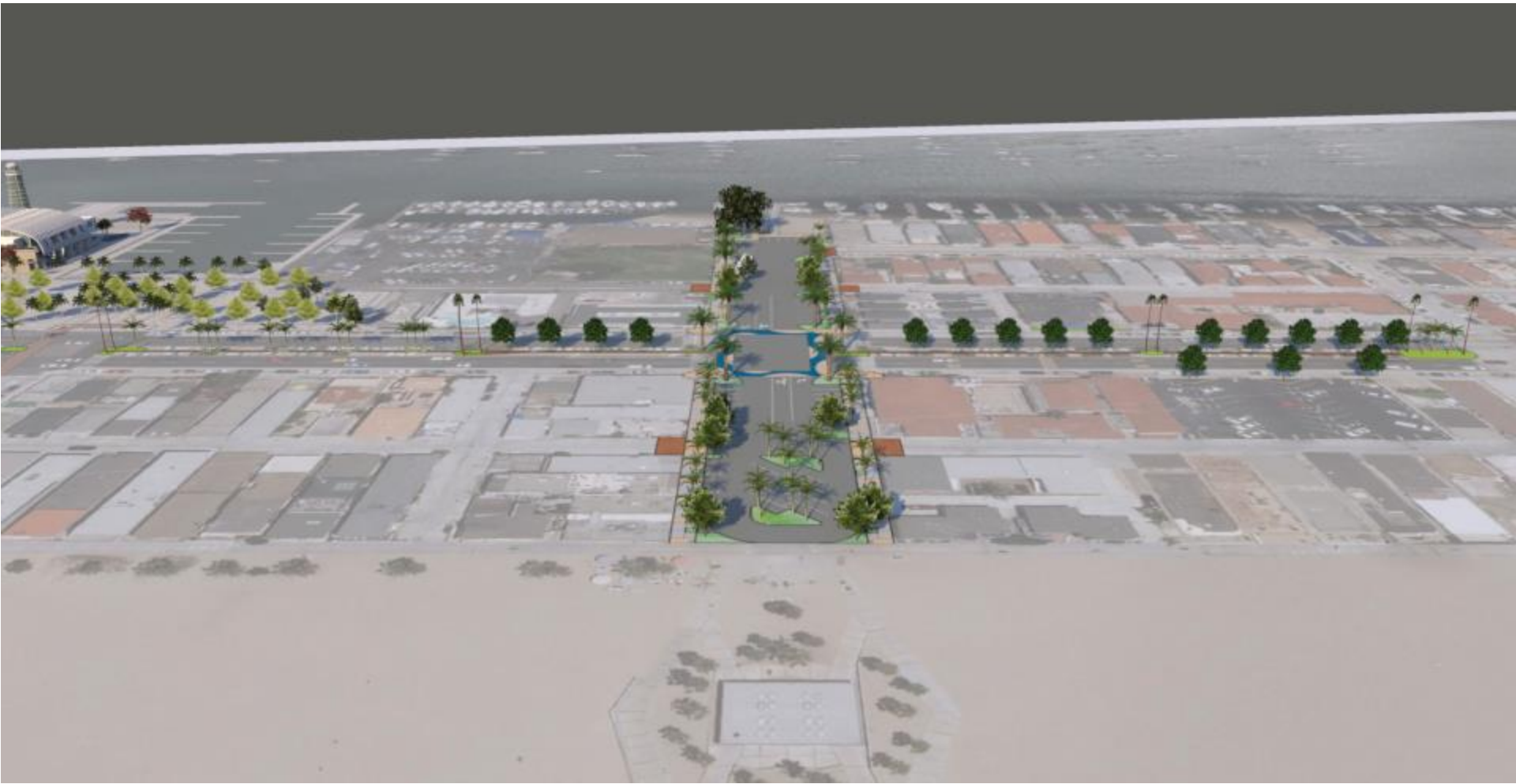
Aerial view of W. Balboa Blvd., 16 th Street to 14 th Street
