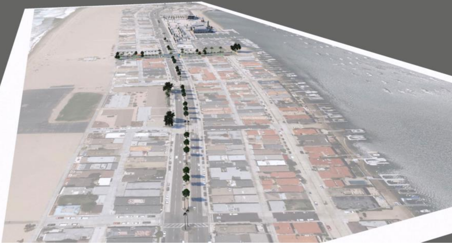
Aerial view looking west down W. Balboa Blvd. Existing Condition shown with proposed Marina Park and 15 th Street Improvements
