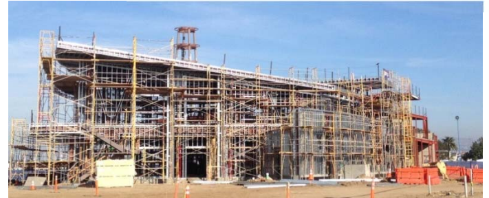
Exterior framing of the Community Center
