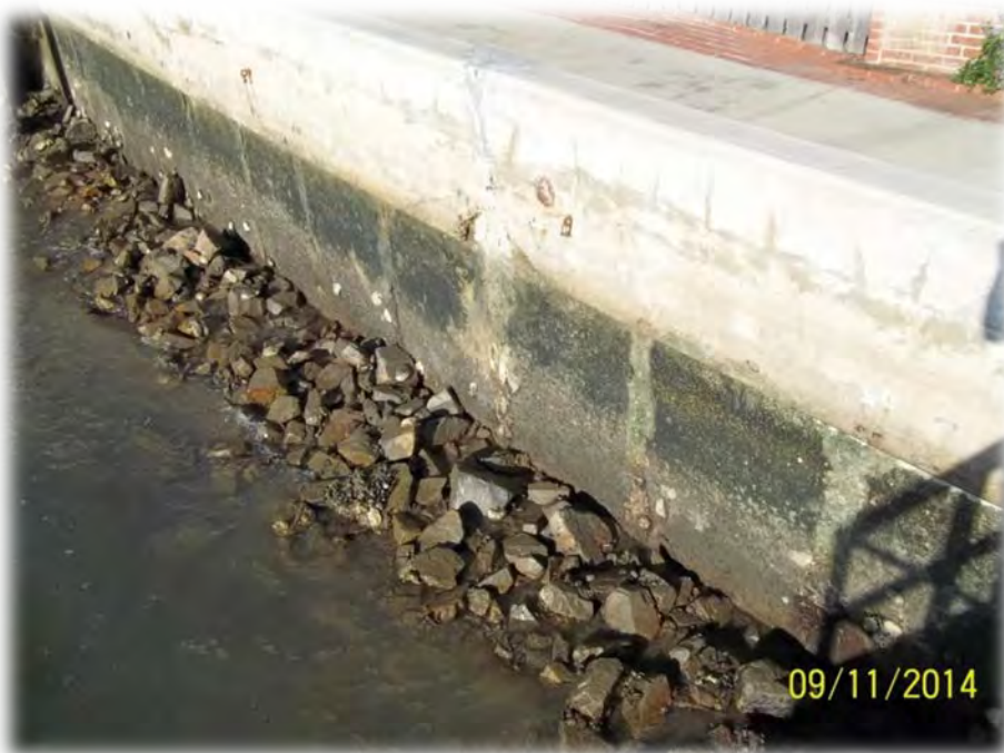
Rock Ballast Placed at West End for Support (1985)
