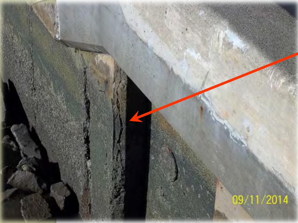
Pile Cracks (West End)
