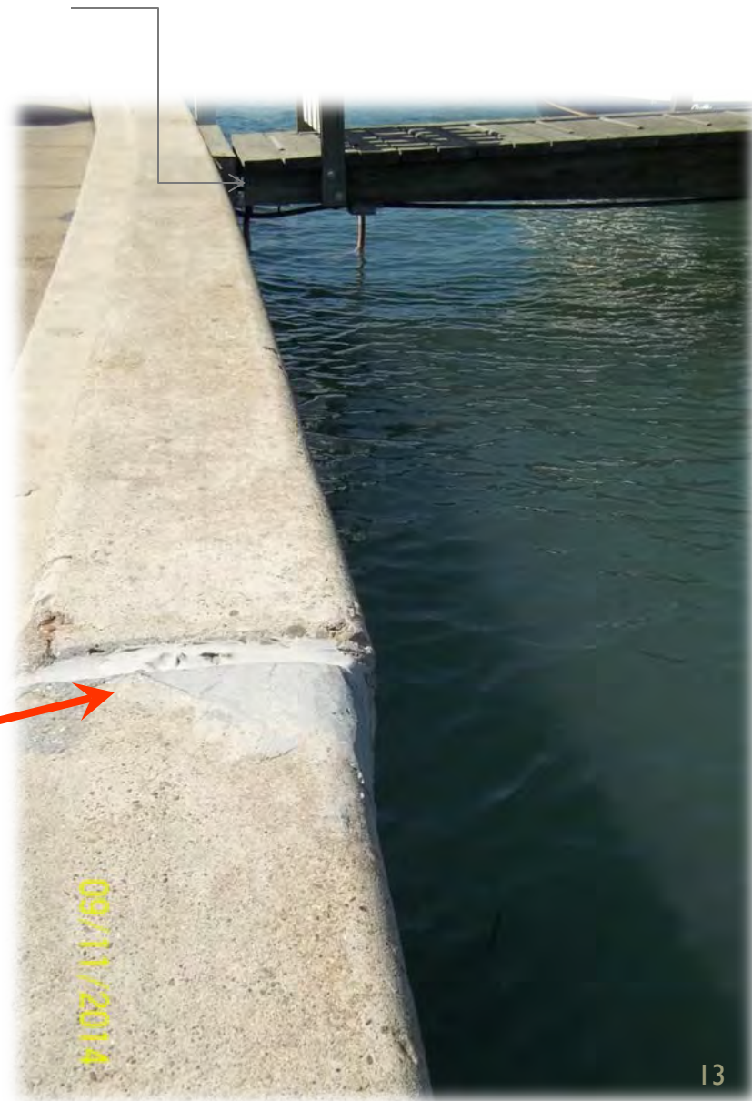
Pile Cracks (West End)
