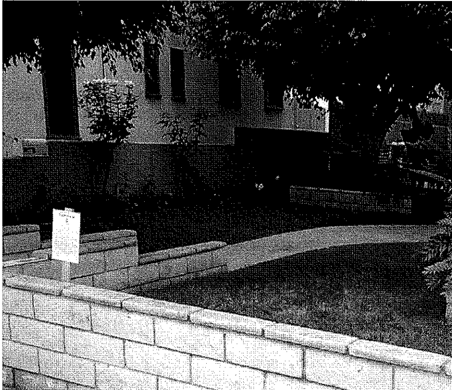
1115 West Balboa Pony Walls, Eastern Side Yard
