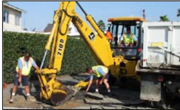
Concrete Maintenance Crew
