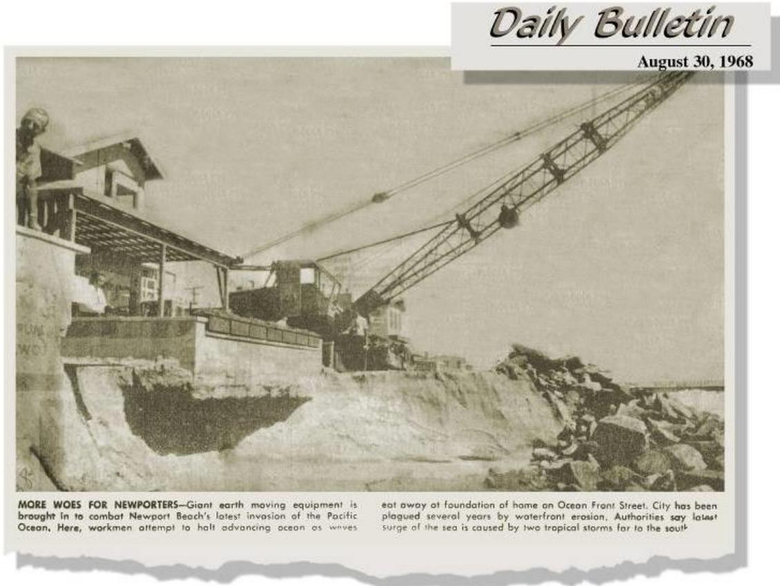
Figure 2-9: Emergency Rip Rap Being Placed at West Newport in August of 1968
