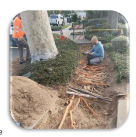
removed without impacting the stability of the trees. The City's tree trimming contractor, Great Scott Tree Service (Great Scott), not only performed the air-spading but also carefully pruned smaller roots identified by Dudek. After this exploratory work was completed, the soil was placed back, and a temporary asphalt patch was installed in preparation of the additional future construction.
