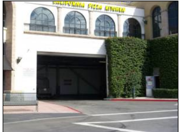
Fashion Island loading dock
