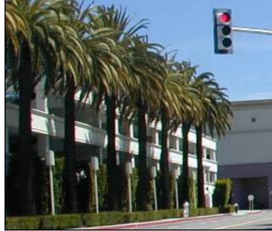
West parking structure at Fashion Island demonstrating rectangular form and varied landscape to soften visual impact
