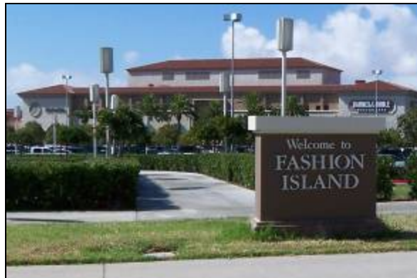
Well-defined walkway from Newport Center Drive into Fashion Island at San Nicolas
