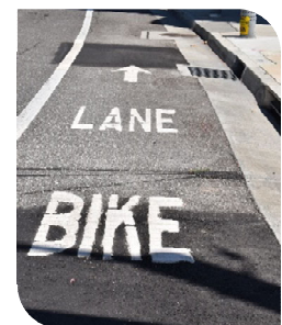
Bicycle Lane, Caltrans Class II
