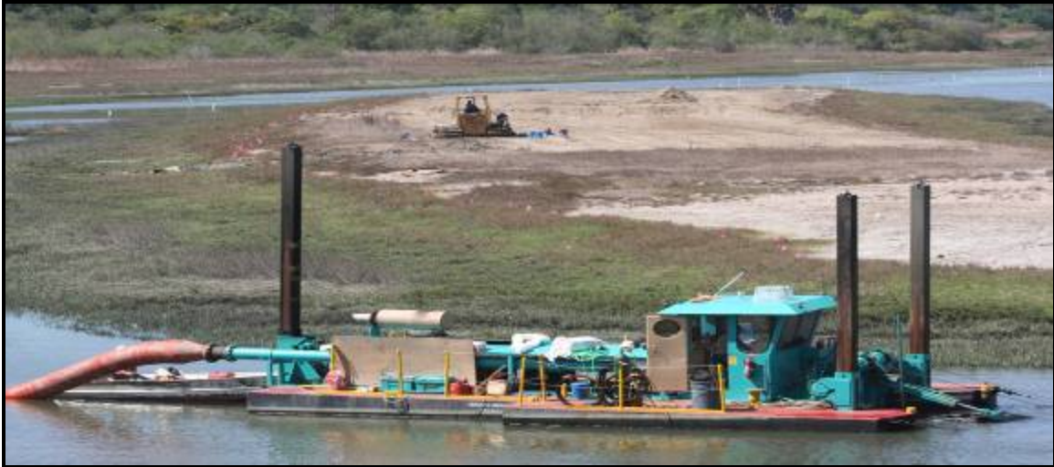
Dredging Hotdog Tern Island Restoration Channel and resurfacing Hotdog Island, Photo by Keane Biological, March 2007
