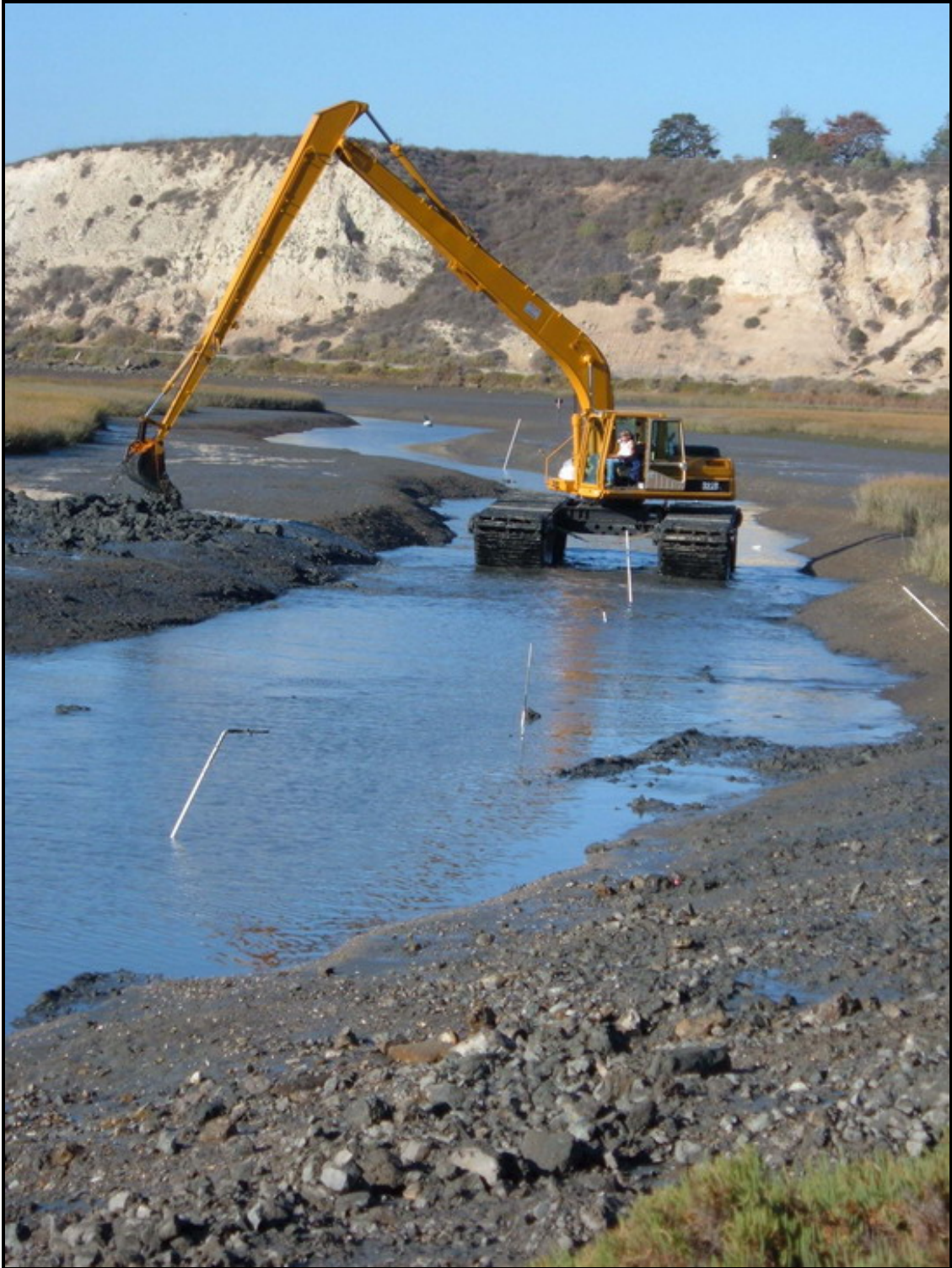
Amphibious Excavator working in Shellmaker Island, October 2008
