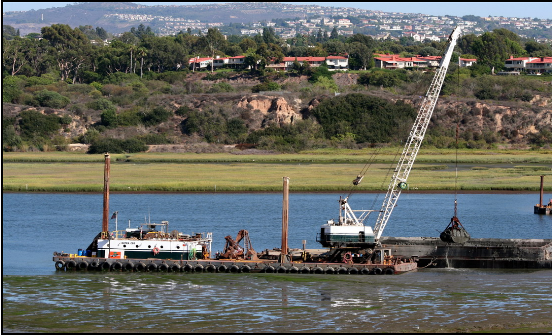
DB-3 dredging Unit II Sediment Control Basin, 29 August 2007
