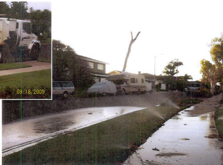
Figure 2. Sprinklers overshooting lawn onto street
