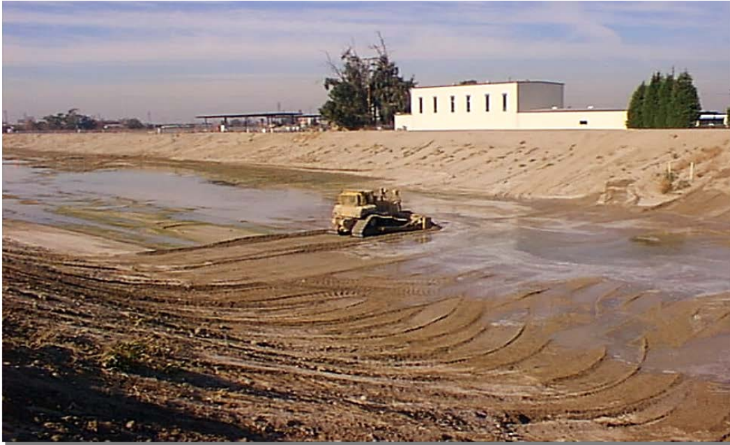
Figure 5-13: Bulldozer in Off-River Channel Removing Clogging Layer
