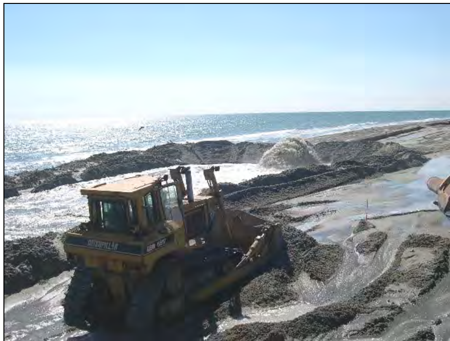
Figure 2. Beach Nourishment Using Dredged Material from Inlet Realignment Project, Emerald Isle, NC
