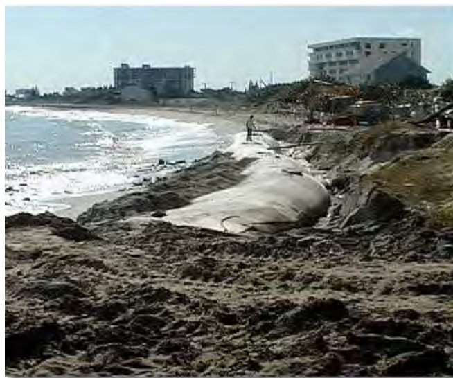
Figure 3. Dredging Material Hydraulically Placed in Geotubes for Shoreline Protection in Atlantic City, NJ
