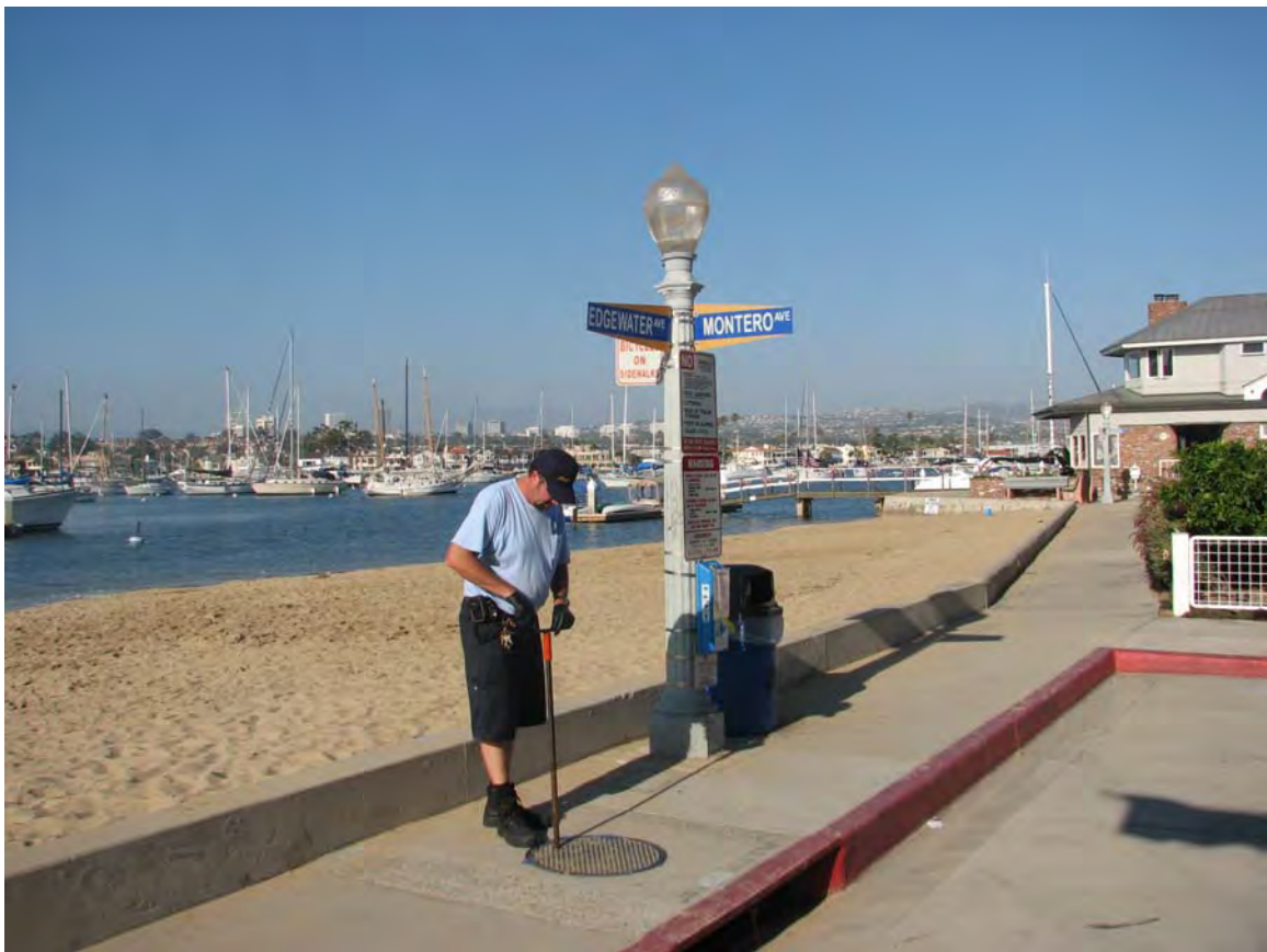
Figure 4.4. General Services staff is responsible for closing 86 tide valves such as this one that prevent bay water from back-flooding the Harbor area during high tides. Once the tide has receded, the tide valve is opened again to permit drainage.
