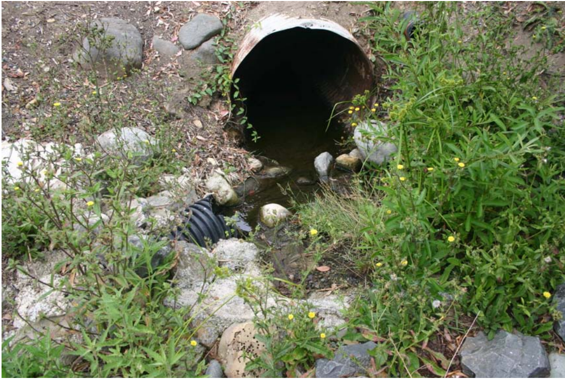
PHOTOGRAPH 1: View of 36-inch pipe discharging to 12-inch pipe at northern end of relict drainage feature.
