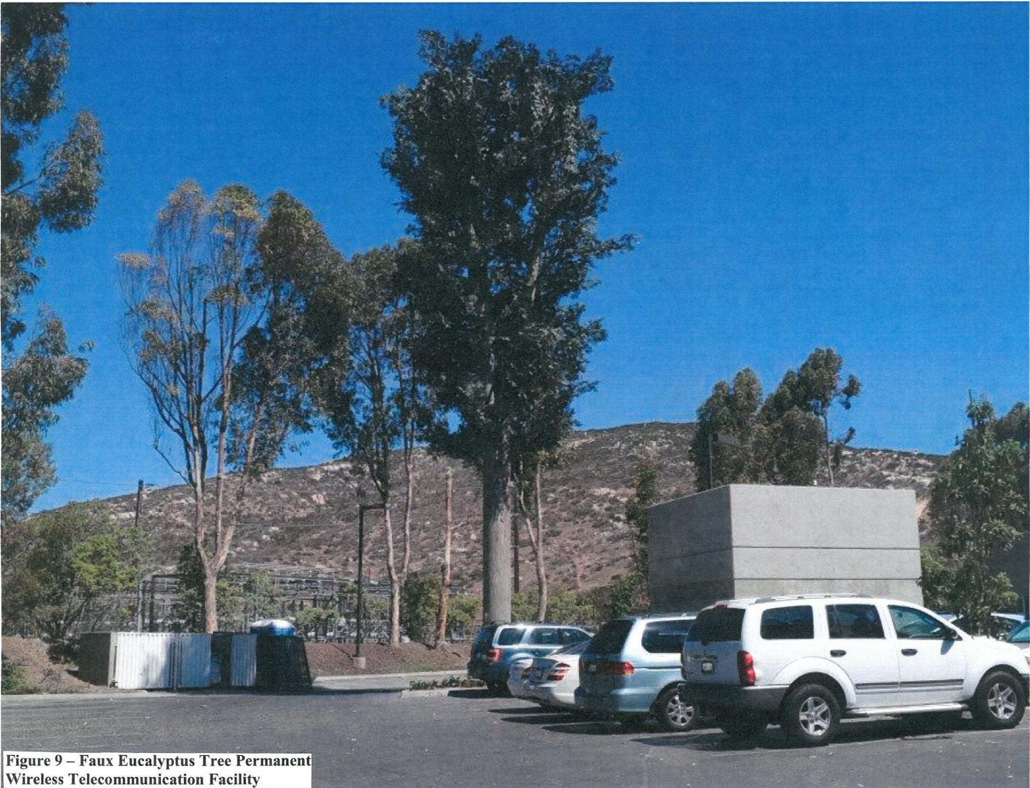
**Figure 9 – Faux Eucalyptus Tree Permanent Wireless Telecommunication Facility**
