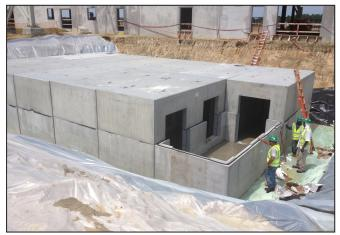
StormCapture detention system installed beneath office parking lot.
