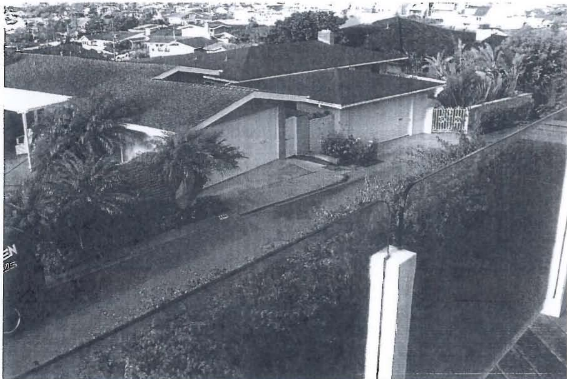
440 Mendoza Terrace Rear deck looking west
