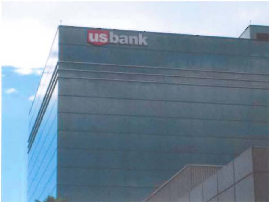
Sign on Dolphinstriker side of subject building.
