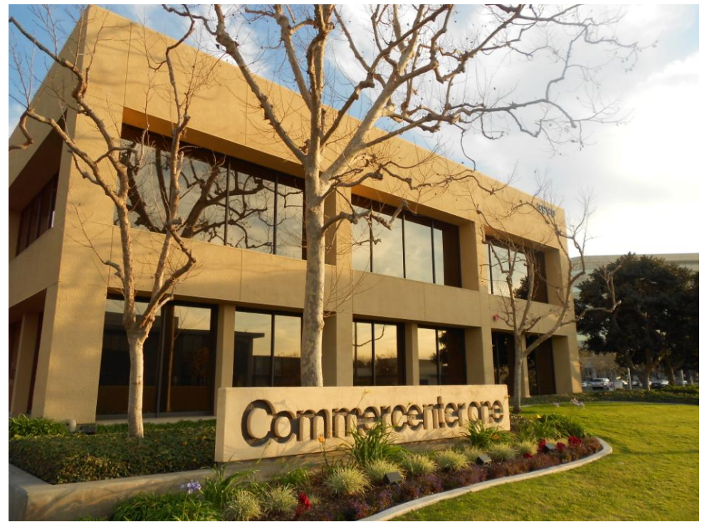
3990 Westerly Place-Westerly Place frontage
