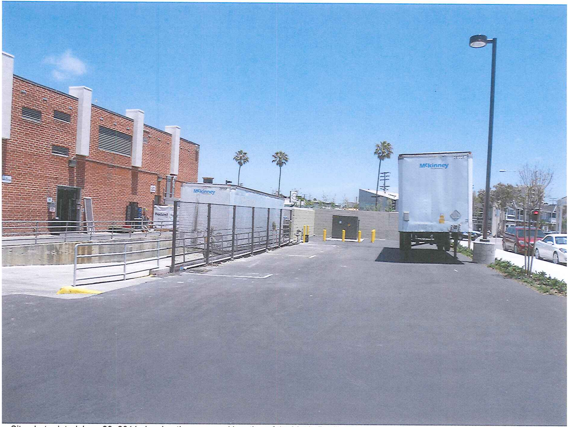
Site photo dated June 29, 2011 showing the proposed location of the Von's Pavilion's temporary refrigeration trailer.
