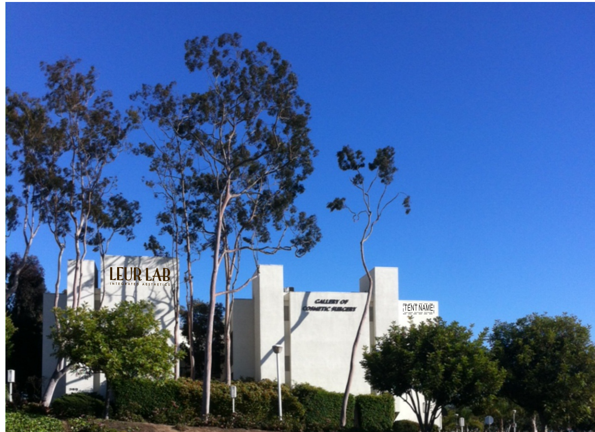
PRIMARY FRONTAGE 359 SAN MIGUEL DRIVEWAY
