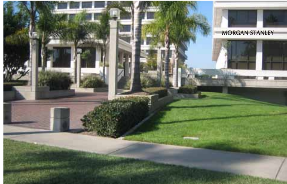
ST 6.7 - VIEW FROM NEWPORT CENTER DRIVE - BUILDING 800
