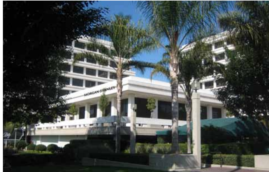
ST 6.6 - VIEW FROM NEWPORT CENTER DRIVE - BUILDING 860/880
