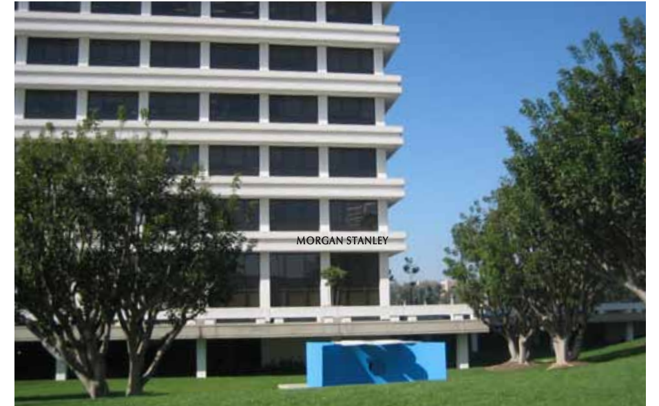
ST 6.8 - VIEW FROM NEWPORT CENTER DRIVE - BUILDING 800
