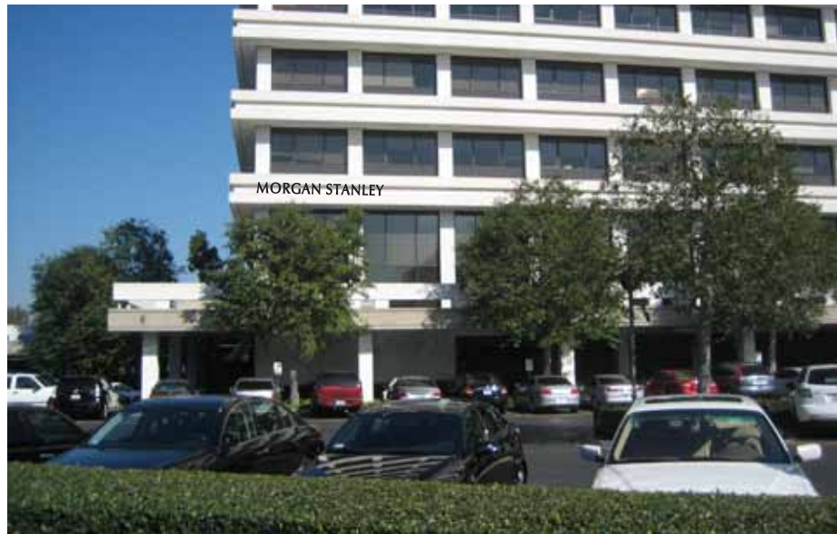
ST 6.1 - VIEW FROM SANTA BARBARA DRIVE - BUILDING 840
