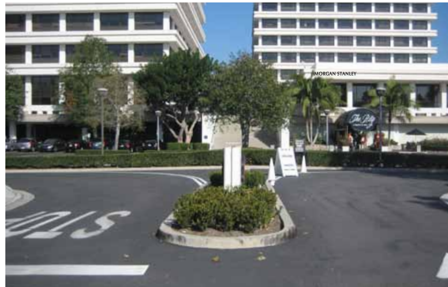
ST 6.3 - VIEW FROM SANTA BARBARA DRIVE - BUILDING 860/880
