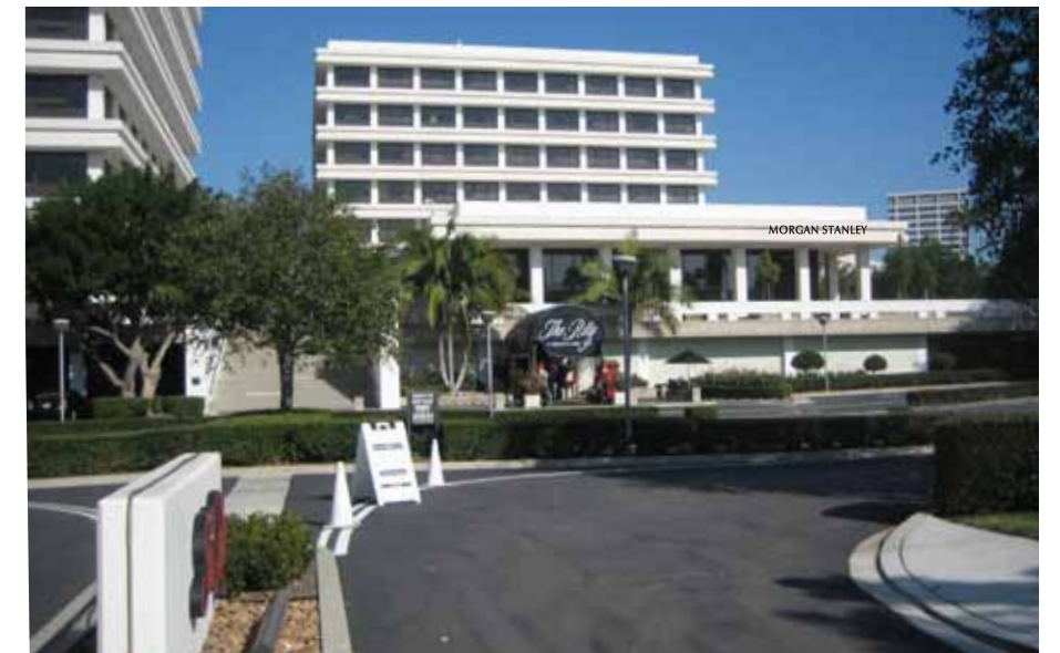
ST 6.4 - VIEW FROM SANTA BARBARA DRIVE - BUILDING 860/880
