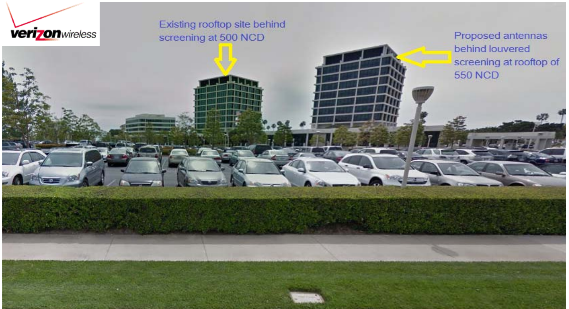
VIEW FROM WEST: Verizon Wireless "Newport Center Relo" – 550 Newport Center Drive
