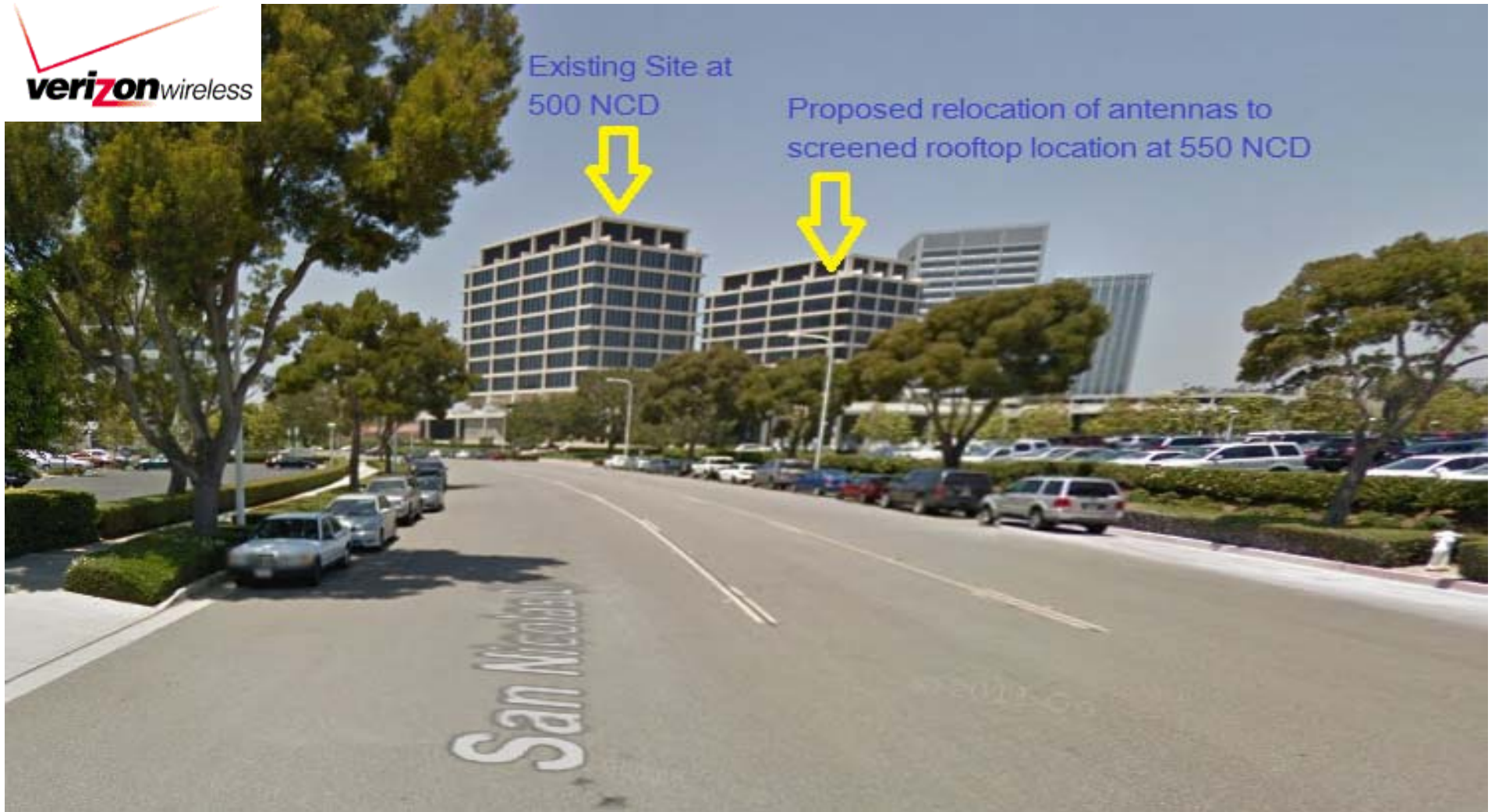
VIEW FROM SOUTH: Verizon Wireless “Newport Center Relo” – 550 Newport Center Drive
