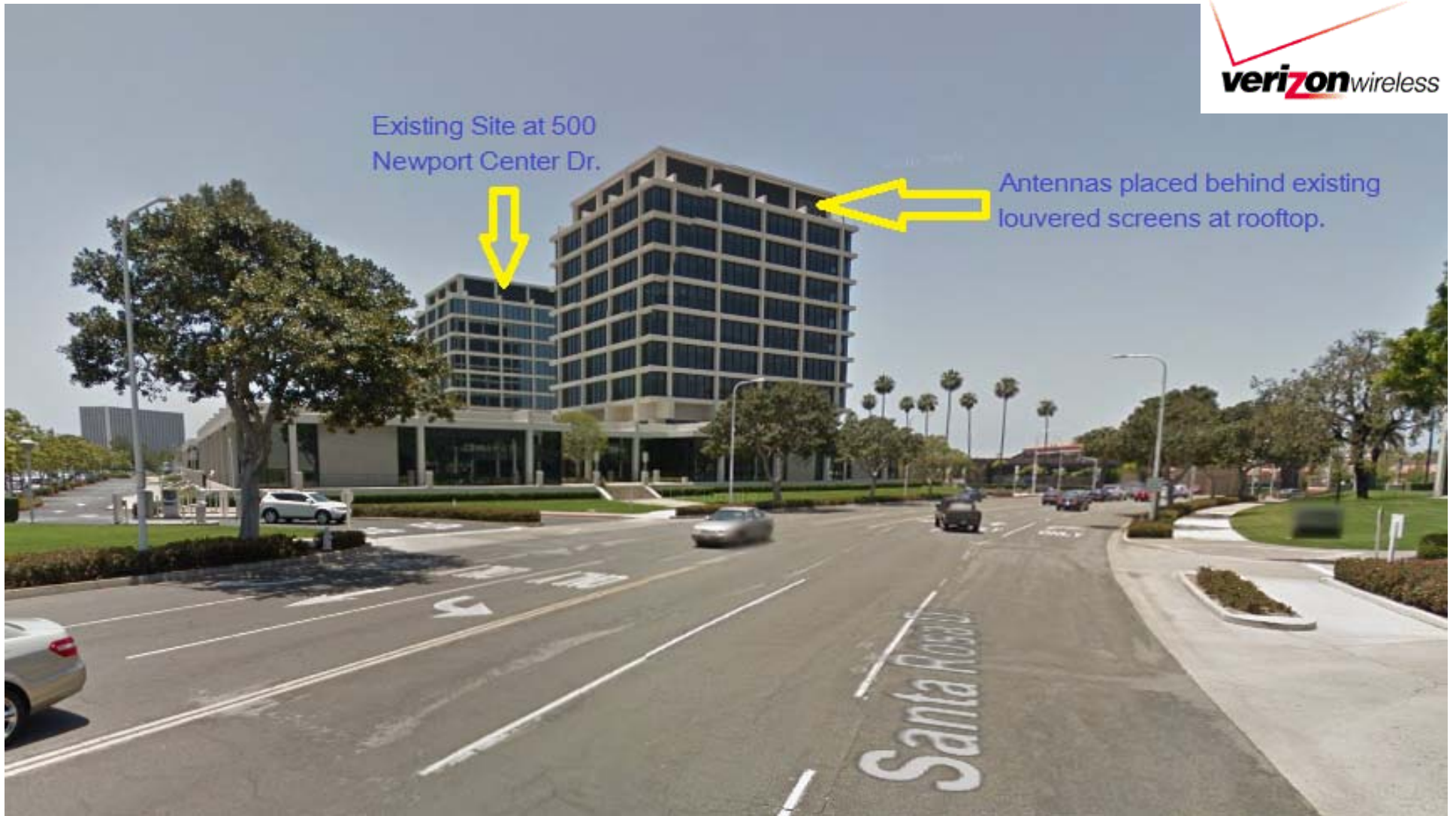
VIEW FROM NORTH: Verizon Wireless "Newport Center Relo" – 550 Newport Center Drive
